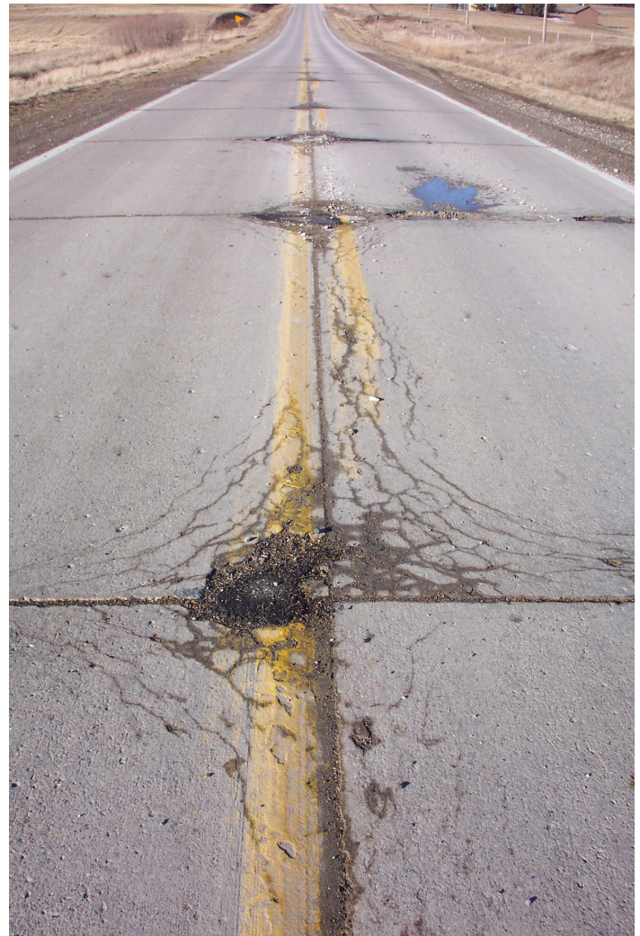
D-cracking on a pavement surface
