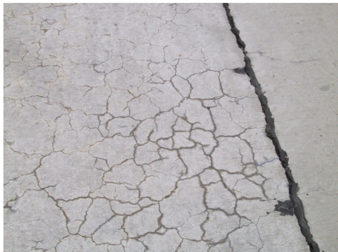
Alkali-silica reaction cracks in a concrete pavement
