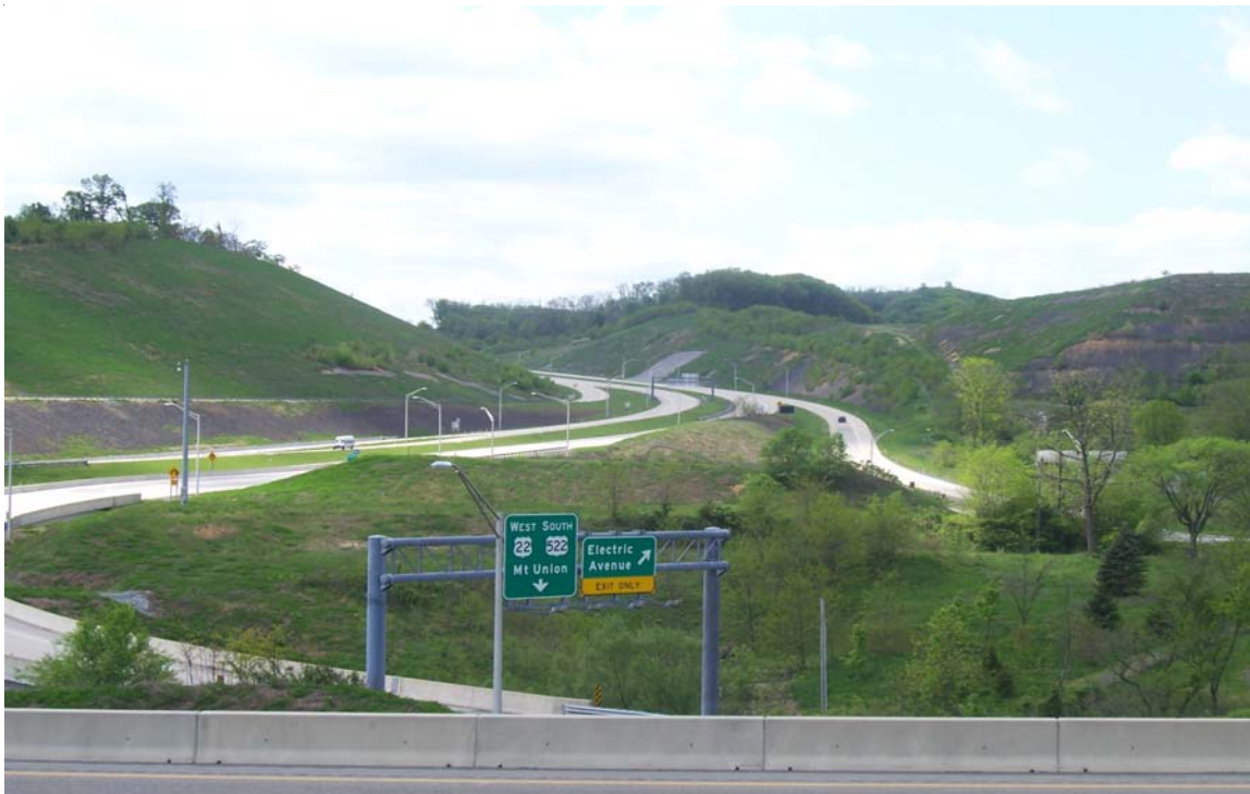
Electric Avenue Interchange near Lewistown
