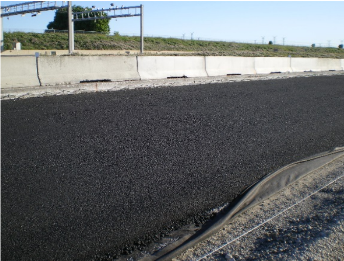
Figure 6. Photo. Asphalt-treated base.
