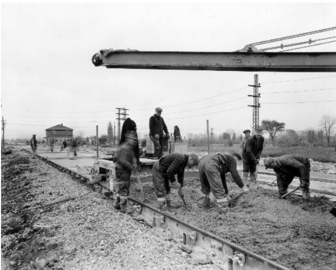
Figure 3. Photo. Early concrete pavement construction in Québec.
