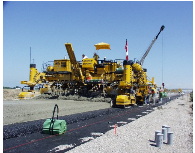
Figure 8. Photo. Base extended beyond the concrete pavement to provide support for the paving equipment.
