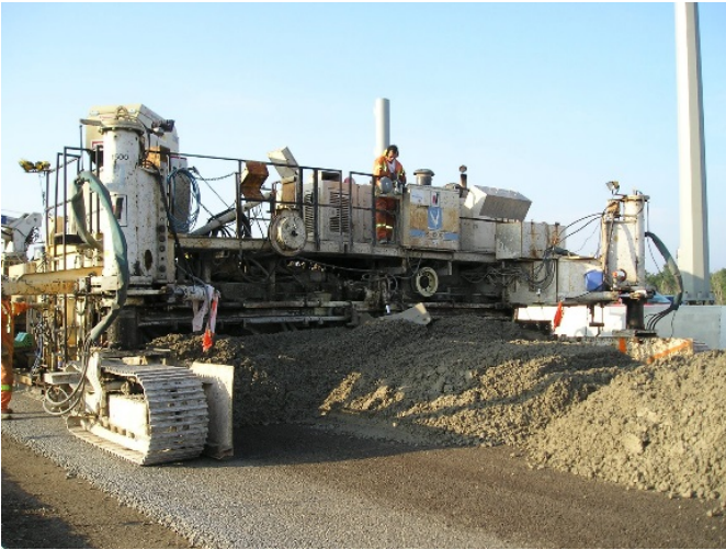
Figure 7. Photo. Cement-treated open-grade drainage layer.
