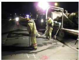
Figure 22. Photo. Grout application into the bottom dowel slots.
