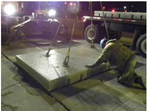
Figure 21. Photo. A typical panel placement.
