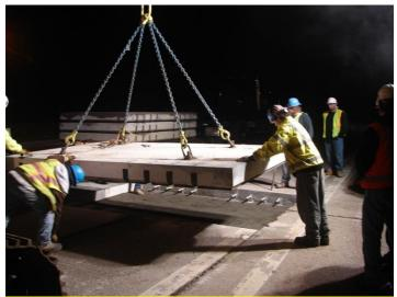
Figure 7. Photo. Super Slab system panel installation.
