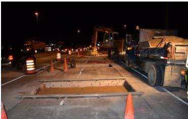
Figure 16. Photo. Distressed slab removal process.
