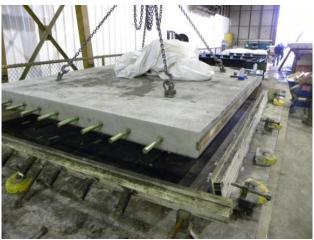
Figure 4. Photo. Super Slab panel form stripping.
