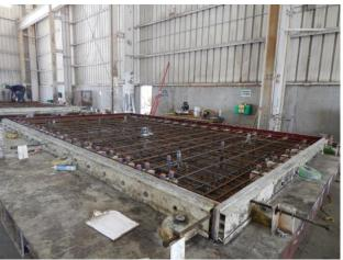
Figure 3. Photo. Super Slab panel form setup.
