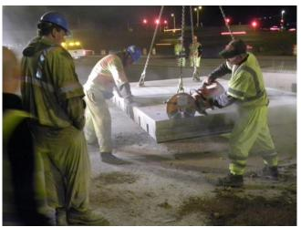
Figure 20. Photo. Panel trimming operation.
