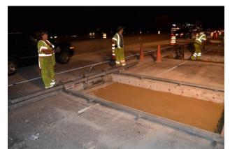
Figure 18. Photo. Fine-grading of the bedding layer.
