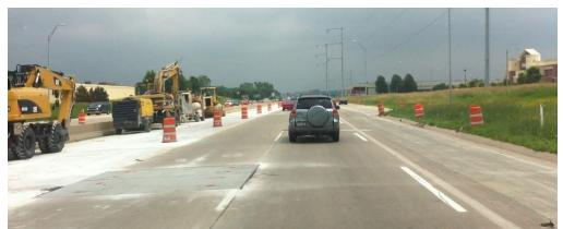
Figure 11. Photo. Stage 2 lane closure and traffic flow after completed repairs in Lane 1 and Lane 2.
