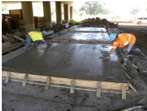
(c) Panel finishing
