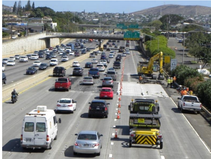
Figure 9. Photo. Daytime closures of lanes 5 and 6.
