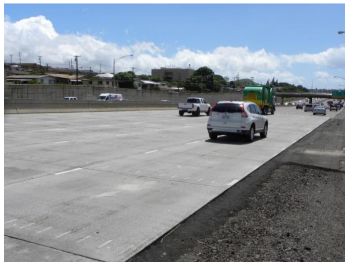
Figure 18. Photo. Completed Hawaii Interstate H1 PCP project.
