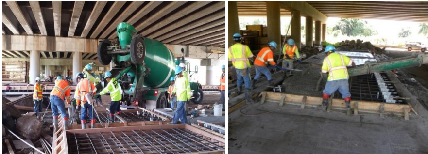
(b) Concrete placement
