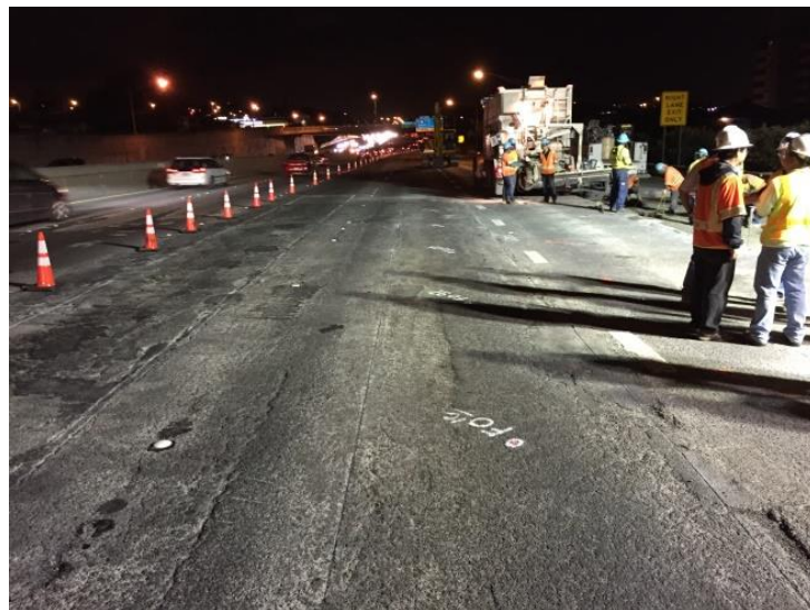
Figure 8. Photos. Typical nighttime lane closures and traffic flow.
