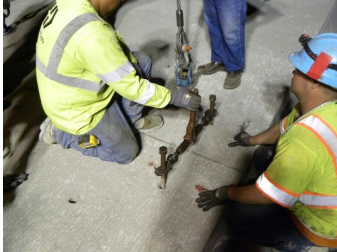
Figure 16. Photo. Turnbuckle use to ensure a tight fit between panels.
