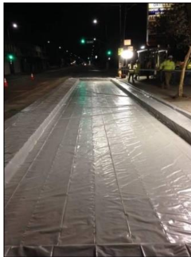
Figure 6. Diagram and photo. The Grout Containment system.
