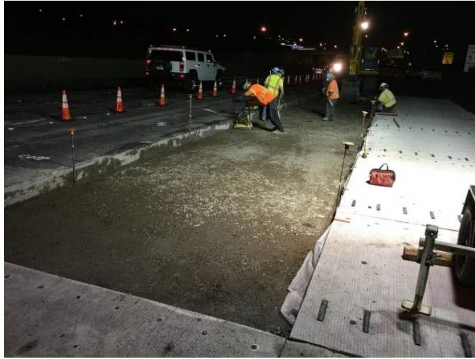
Figure 12. Photo. Existing base grading.
