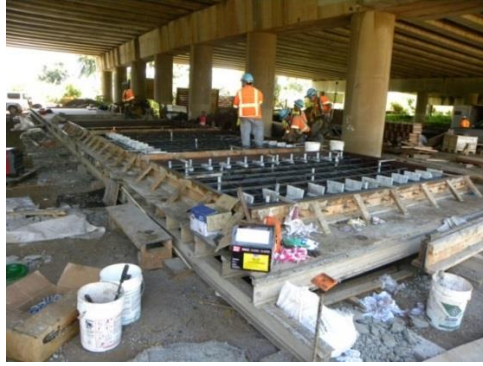
(a) Panel formwork ready for concrete placement
