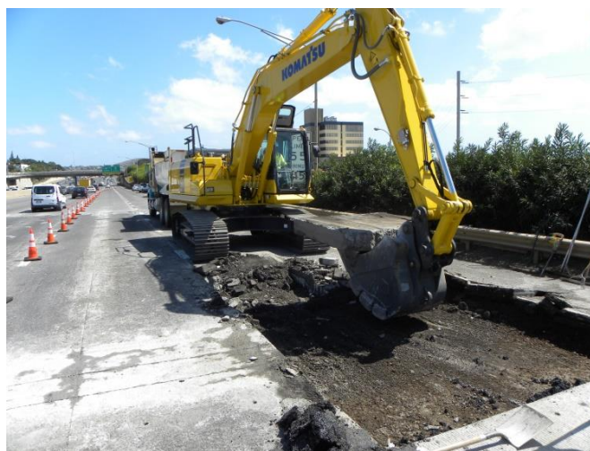
Figure 11. Photo. Existing pavement removal.
