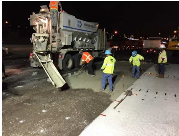
Figure 13. Photo. CTB placement using a mobile mixer.
