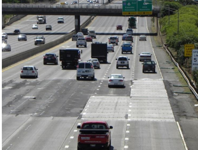
Figure 3. Photo. Lanes 5 and 6 partially replaced with precast panels.
