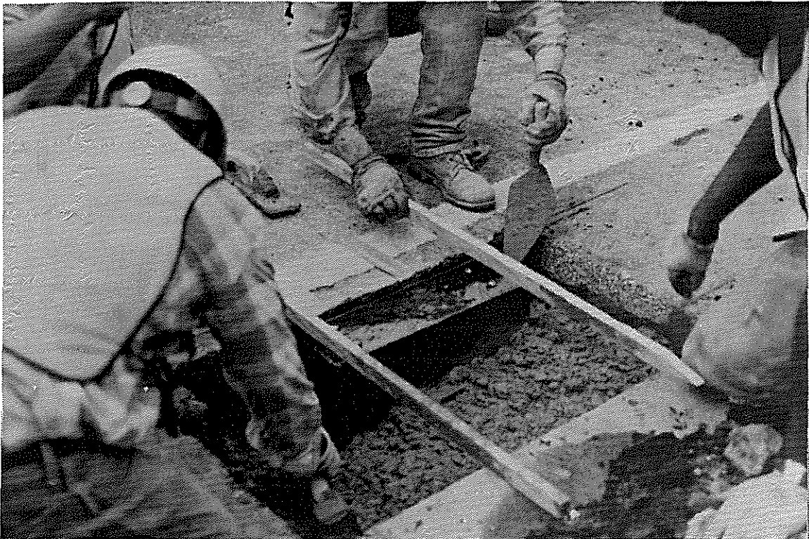
Figure 12. Installation of Utility Box..
