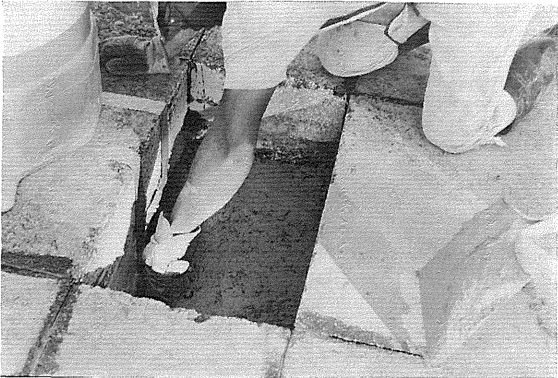
Figure 11. Preparing Base for Utility Box.
