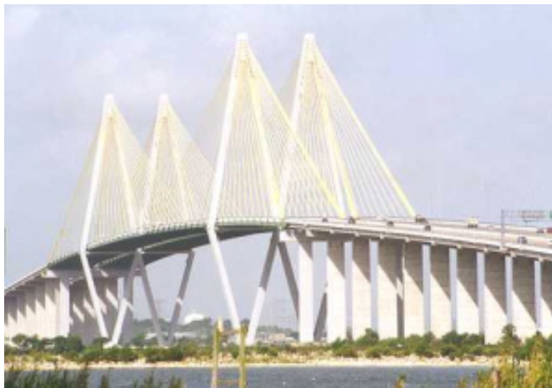
Figure 10: Fred Hartman Bridge.
