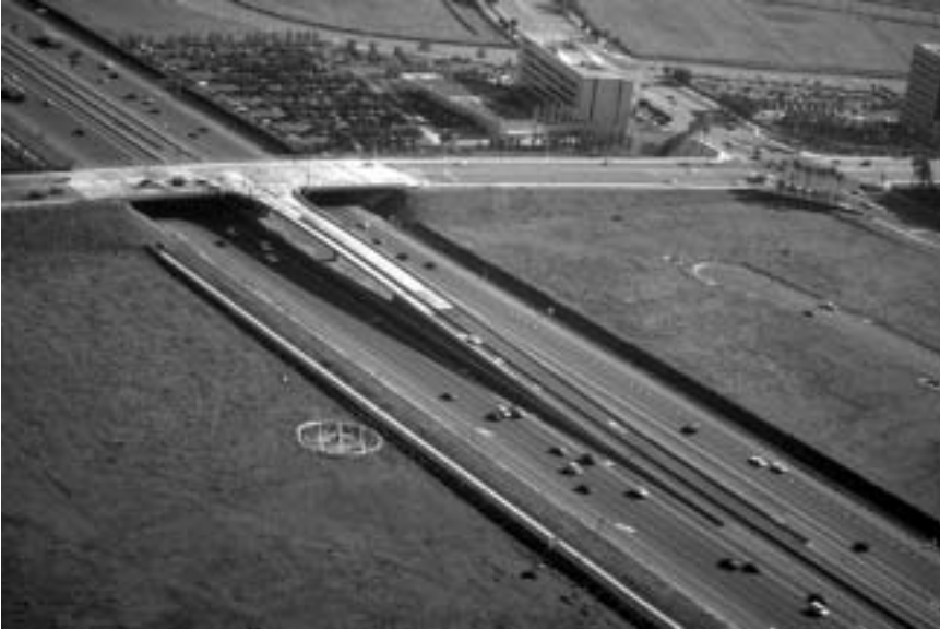
Figure 15. Elevated HOV drop ramp
