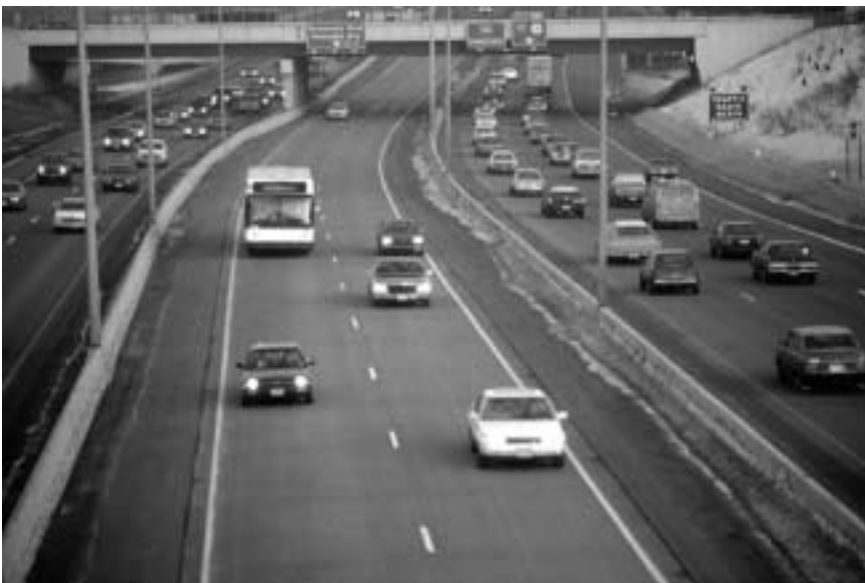
Figure 12. Concrete barrier on I-394 reversible lanes, Minneapolis
