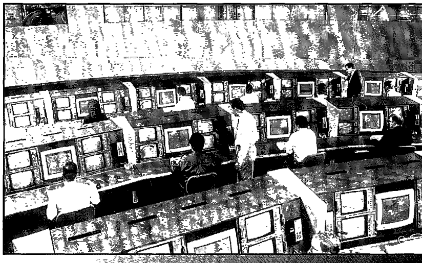
TransGuide Control Center, San Antonio
