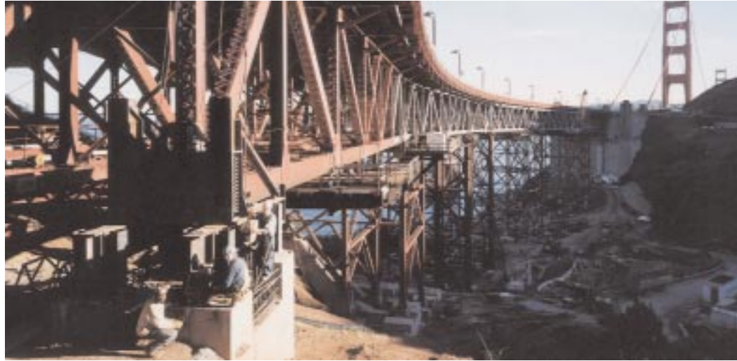
The Golden Gate Bridge is among the go U.S. bridges being retrofitted with seismic isolation systems.
