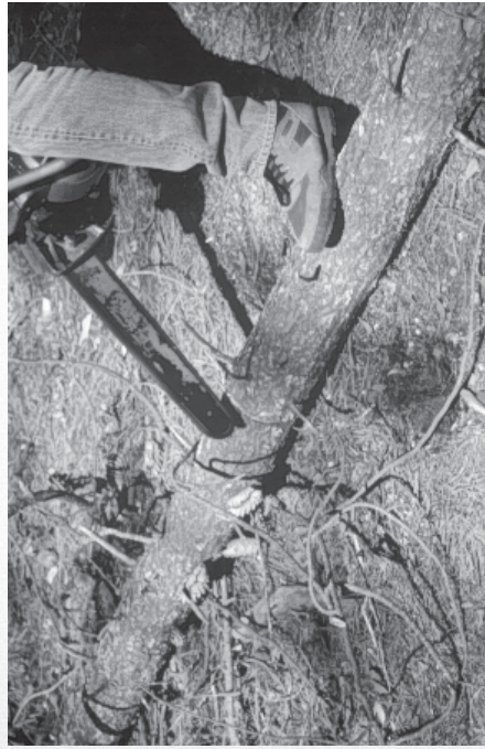
Figure 18-1. Obstacles, such as fallen trees, should be removed to maintain the tread in a condition that can be negotiated by all trail users.
