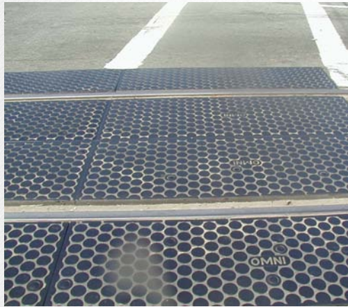
Figure 8-27. Installing a rubber surface rather than asphalt around railroad flangeways reduces changes in level and other maintenance problems for pedestrians.
