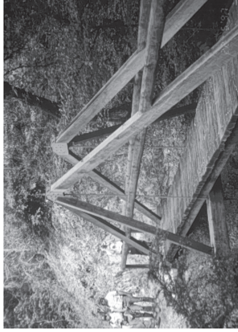
Figure 16-8. GOOD DESIGN: On this outdoor recreation trail, the width of the bridge is consistent with the width of the trail leading up to the bridge.
