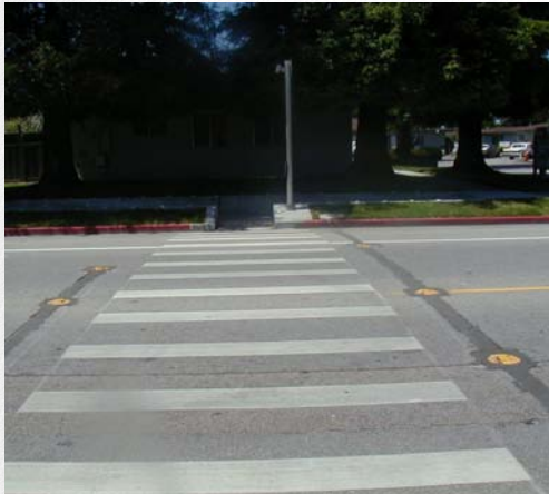
Figure 8-13. Imbedding lights in the asphalt at the edge of a crosswalk is an experimental method for making crosswalks more visible to motorists.
