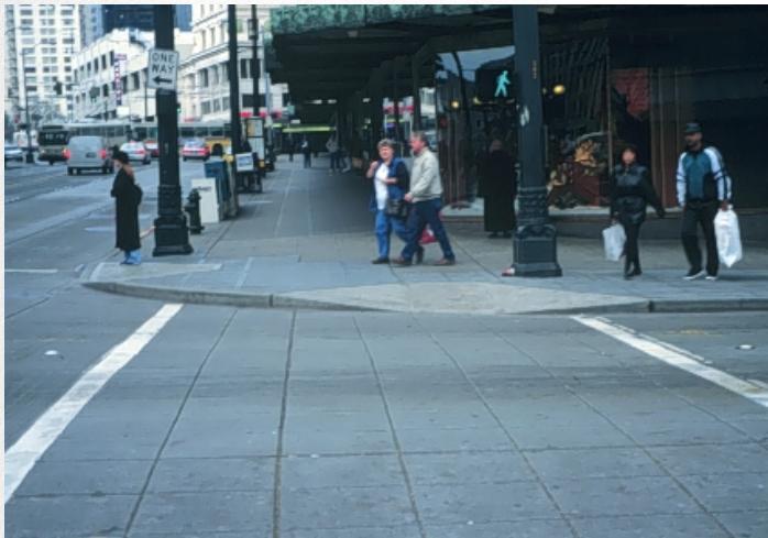
Figure 7-1. Curb ramps should be designed to provide access to people with mobility limitations and vision impairments.
