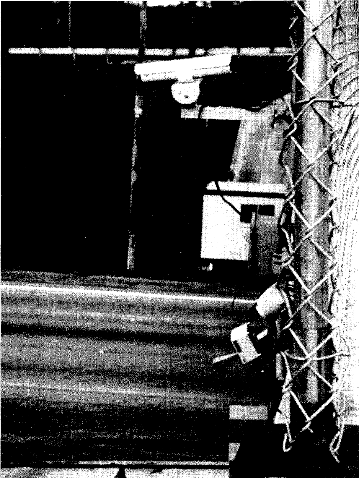
Figure 9-21. View Toward Eastbound I-4 Showing Side-Mounted RTMS Microwave Detector, Trailer, Video Camera, and Overhead Detectors
