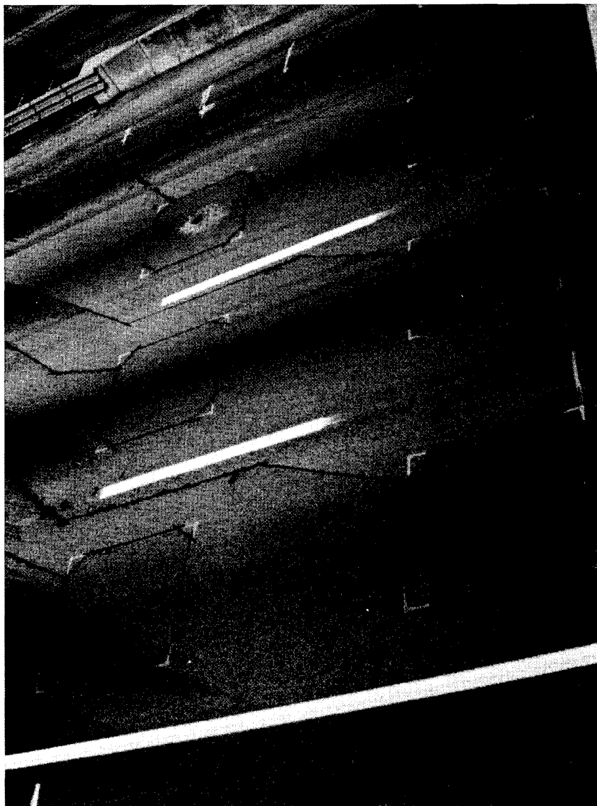
Figure 9-18. I-4 Freeway Lanes Showing Installed Inductive Loops and Self-Powered Magnetometers
