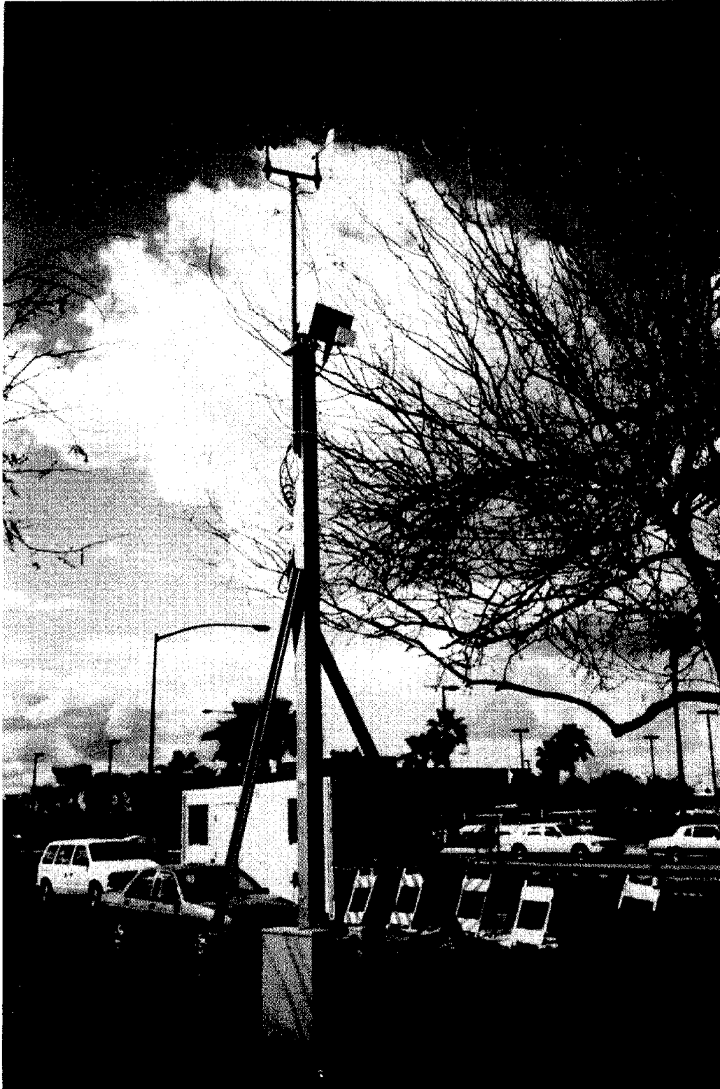
Figure 9-51. Pole-Mounted Wind Speed and Direction Sensors and Side-Viewing RTMS Microwave Detector at Oracle Road Site
