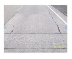
Figure 28. Longitudinal cracking near the shoulder in lowa-0217 section (March 30, 2011).
