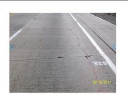
Figure 23. Longitudinal cracking near the shoulder in Arkansas-0213 section (May 24, 2007).
