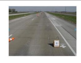
Figure 30. Longitudinal cracking near the shoulder in Washington-0206 section (May 23, 2013).
