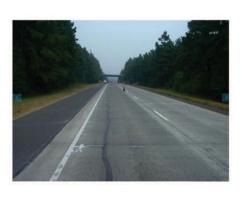
Figure 24. Longitudinal cracking near the shoulder in Arkansas-0217 section (December 4, 2012).
