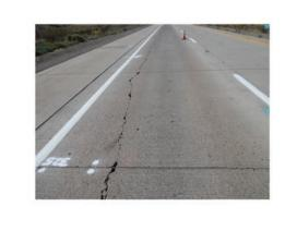
Figure 22. Longitudinal cracking near the shoulder in Arizona-0262 section (February 16, 2011).
