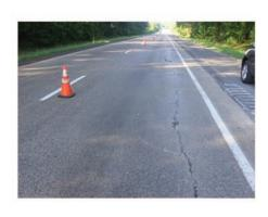
Figure 25. Longitudinal cracking near the shoulder in Colorado-0217 section (September 20, 2011).
