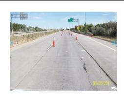
Figure 27. Longitudinal cracking near the shoulder in North Dakota-0217 section (August 21, 2012).
