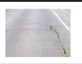
Figure 29. Longitudinal cracking near the shoulder in Ohio-0206 section (September 12, 2006).
