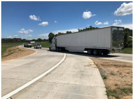
Figure 30. Photo. Completed precast pavement installation.
