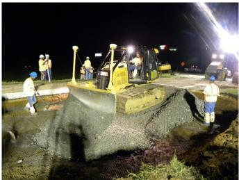
Figure 12. Photo. Ballast aggregate placement.
