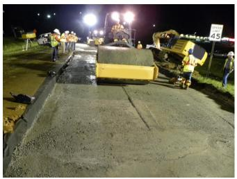
Figure 14. Photo. Base compaction.
