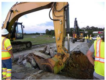
Figure 9. Photo. Broken concrete removal.
