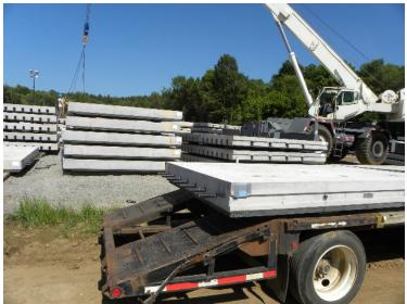
Figure 7. Photo. Staging area for panels.
