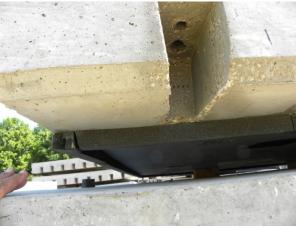
Figure 5. Photo. View of the panel bottom showing gasket around dowel bar slots.
