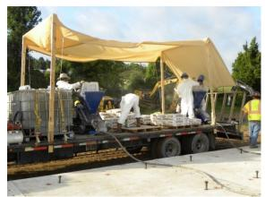
Figure 24. Photo. Two grout mixers used for grouting.
