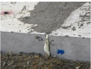
Figure 26. Photo. Polymer foam use at ends of transverse joints to prevent grout leakage.
