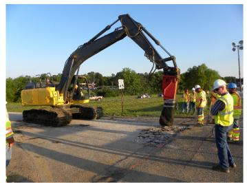
Figure 8. Photo. Existing concrete pavement demolition.
