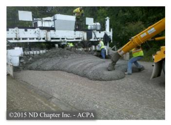
Figure 4. Placement of a 4-inch (102 mm) bonded overlay on a milled asphalt pavement near Devils Lake, ND (NDRMPCA 2015).
