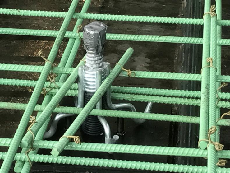
Figure 6. Photo. The leveling lift system placed in the panel formwork.
