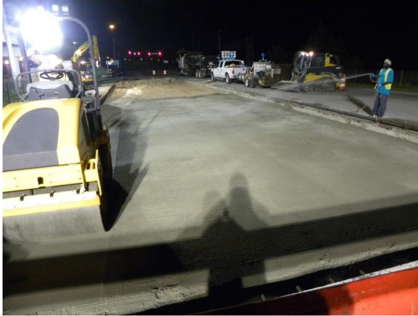
Figure 20. Photo. Compaction and water spraying of the sand-cement layer.
