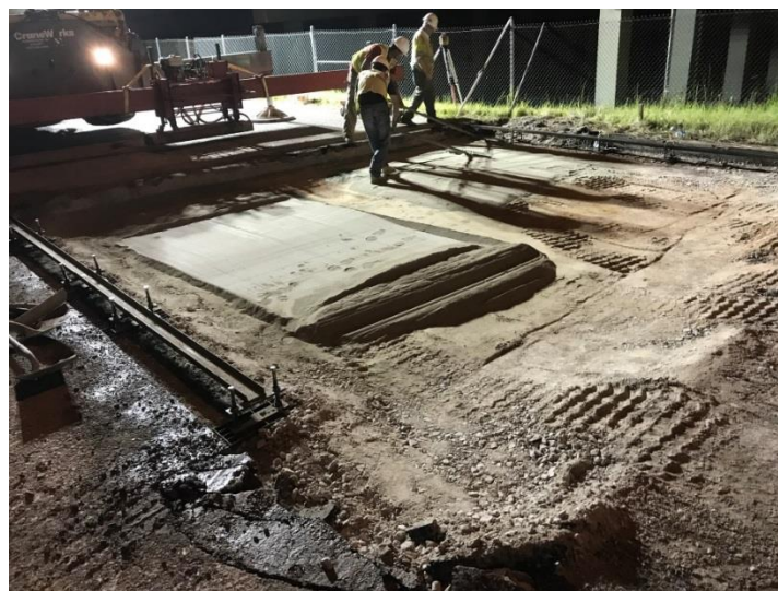
Figure 14. Photo. Placement of the dry sand-cement mixture.
