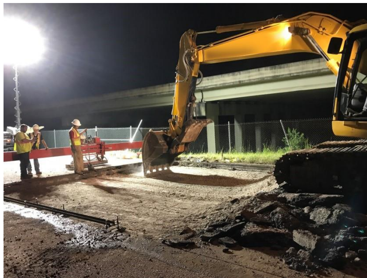
Figure 11. Photo. Excavator trying to scarify the granular base.
