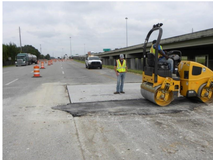
Figure 16. Photo. AC patch at the end of the second precast panel.
