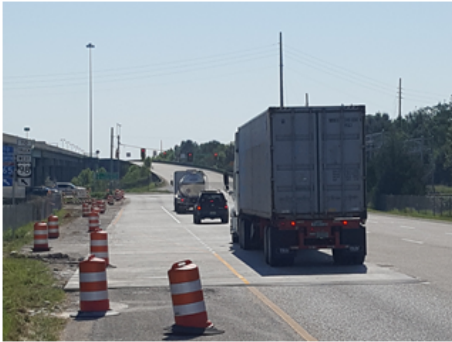
Figure 25. Photo. Completed precast pavement installation.
