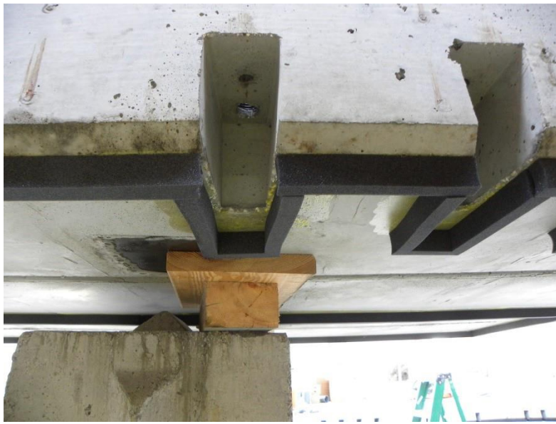
Figure 9. Photo. View of the panel bottom showing gasket around dowel bar slots.
