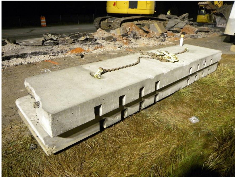
Figure 17. Photo. Dummy panels for use at end of each night's installation.
