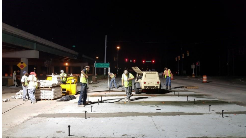
Figure 22. Photo. Using leveling bolts to set panel elevation.
