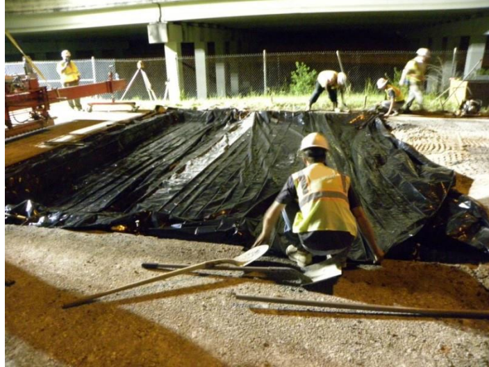
Figure 15. Photo. Covering up of the work area.
