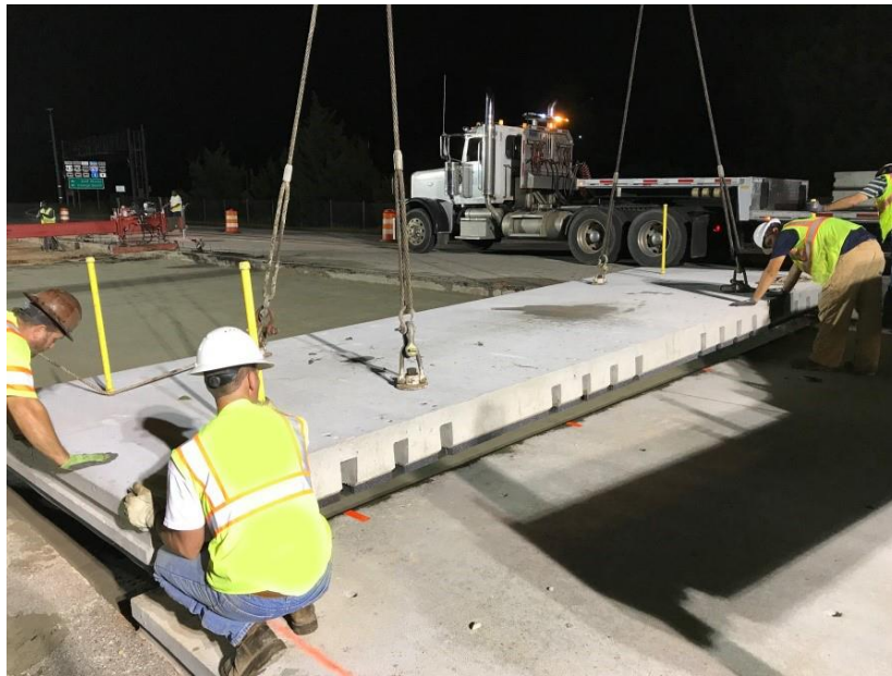
Figure 21. Photo. Placement of a panel.
