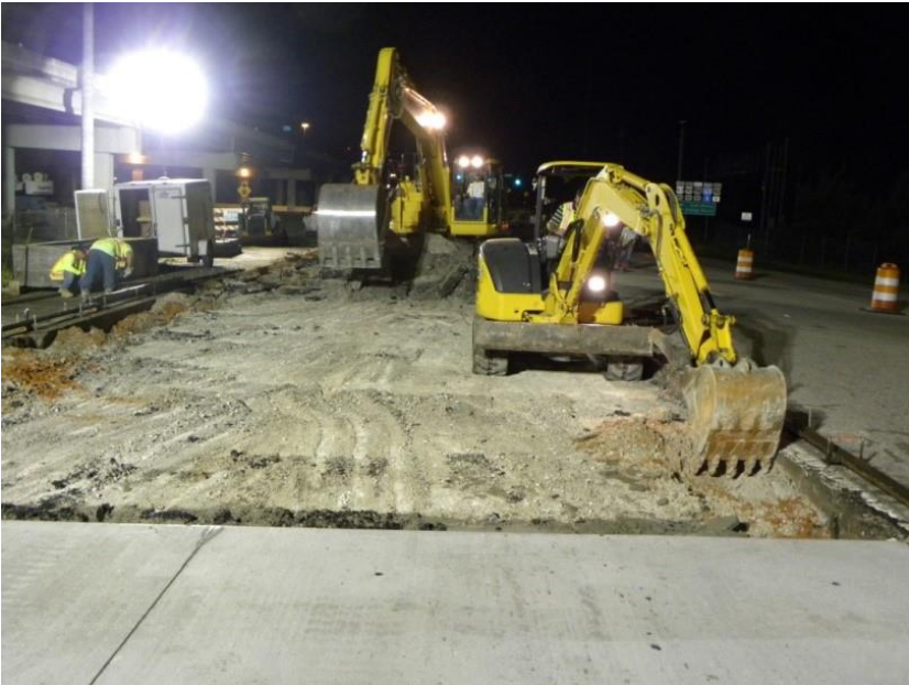
Figure 18. Photo. Base preparation for the production panel installation.
