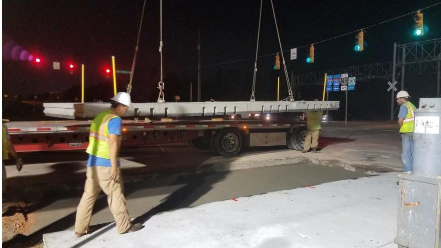
Figure 24. Photo. Last panel being installed at the intersection.
