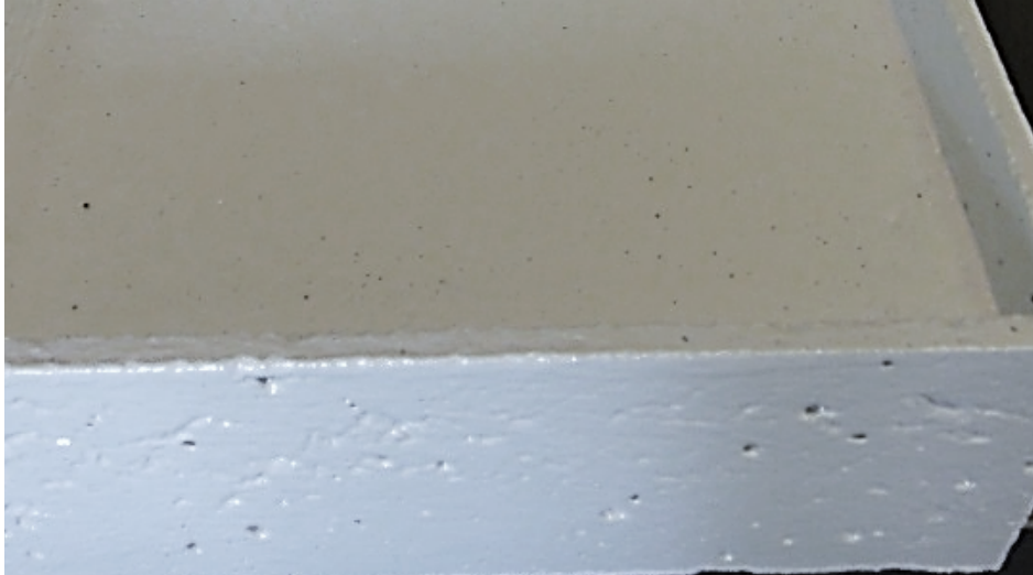
Figure 7. Coated concrete block with pinholes
