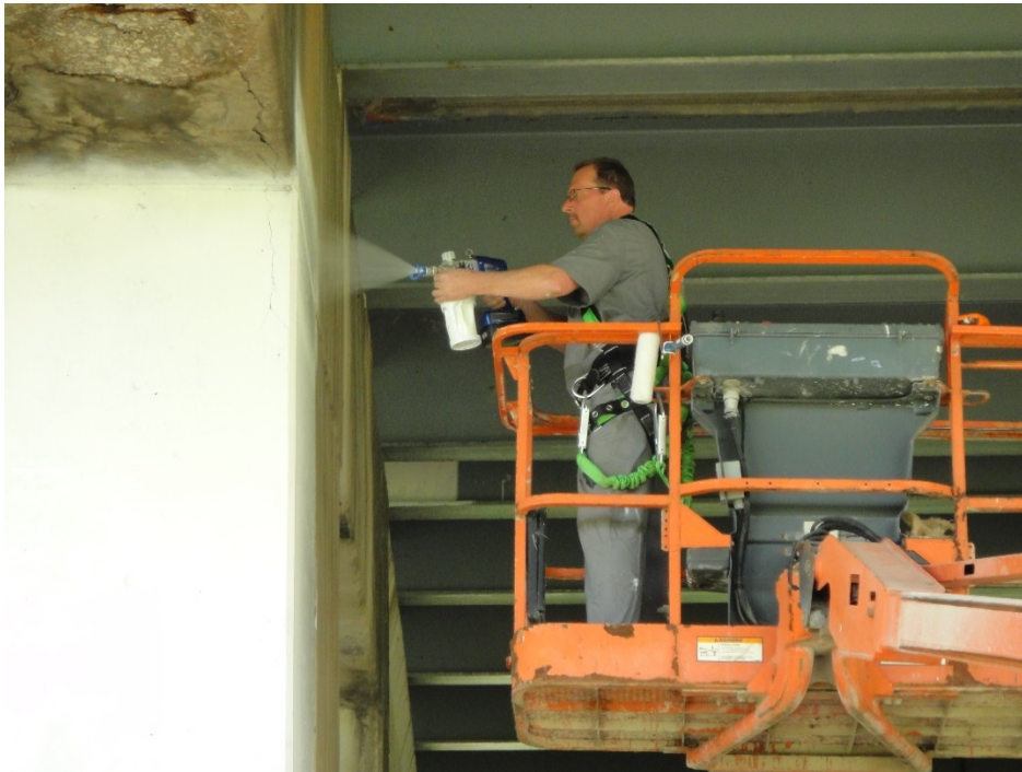
Figure 6. Spray application with a Graco ProShot HD
