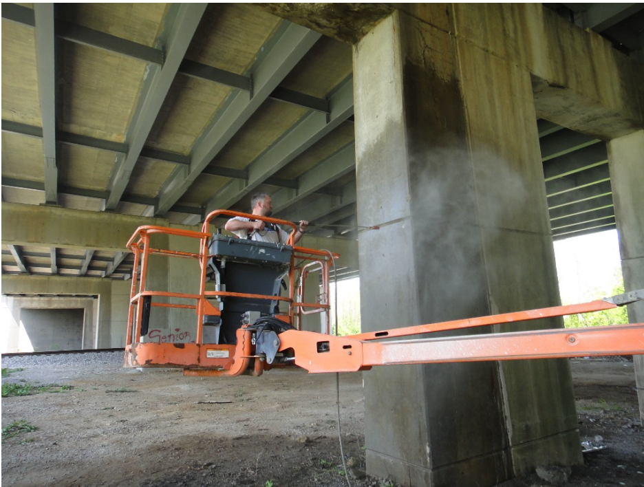
Figure 2. Pressure washing concrete substrate prior to coating.
