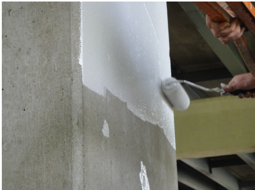
Figure 4. Applying coating to concrete on bridge column
