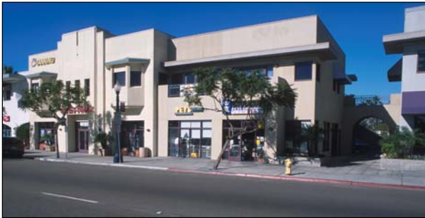
A pedestrian arcade connects a bus stop on University Avenue to the core of the neighborhood.
