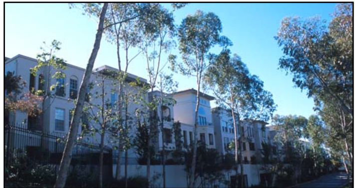
The ‘Uptown District’ in San Diego is an example of how bus TODs can be part of a community’s strategy to
