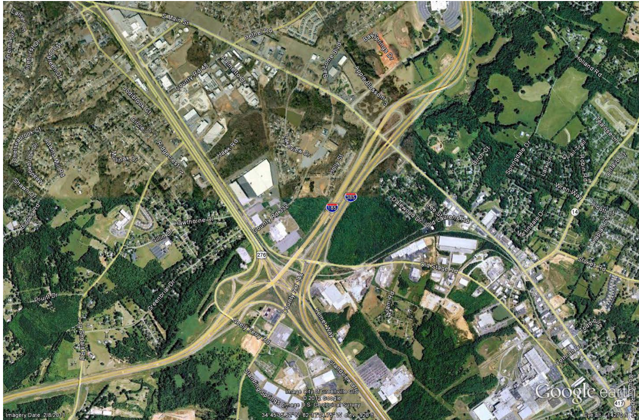
Figure 79. Photo. Configuration of site SC-2. (49)
