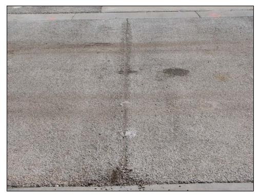
FIGURE D-6: Tooled joint, 4.02.09.
