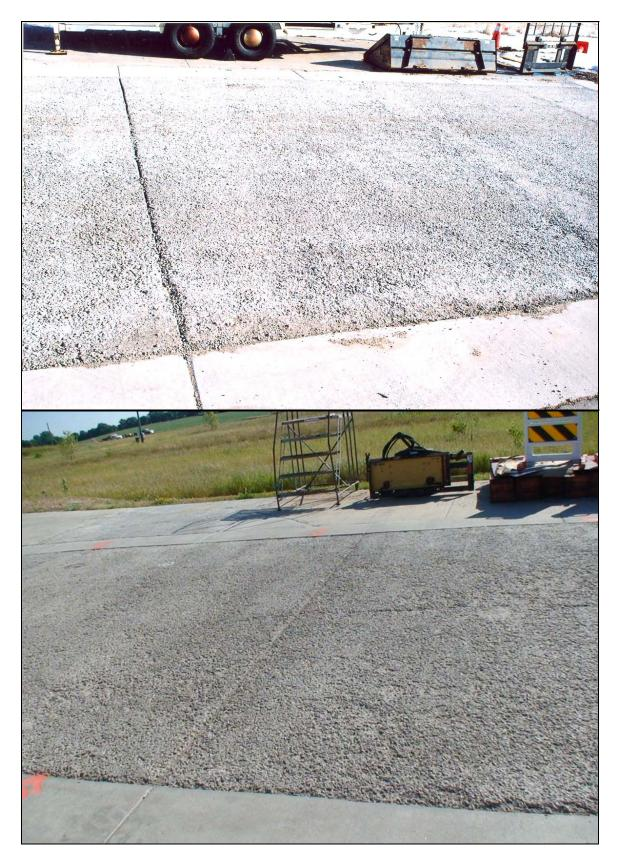
FIGURE D-2: Header/construction joint, Top: 9.21.06, Bottom: 8.11.08.
