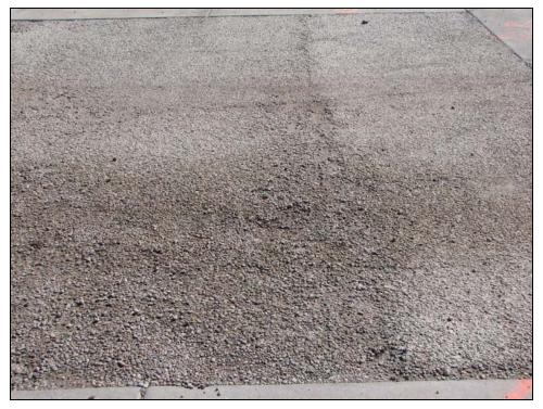
FIGURE D-7: Area of severe raveling in Mix 2, 4.02.09.
