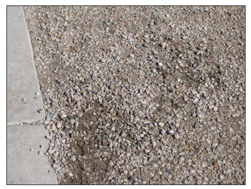
FIGURE D-8: Raveled surface material in Mix 2, 4.02.09.
