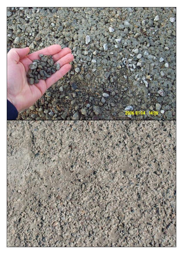
FIGURE D-3: Mix #2 surface raveling, Top: 01.04.06, Bottom: 8.11.08.
