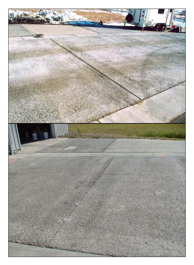
FIGURE D-1: Tooled joint, Top: 9.21.06, Bottom: 8.11.08.
