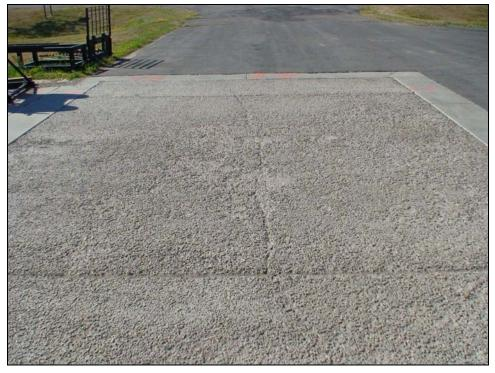
FIGURE D-5: Header/construction joint, facing south, 8.11.08.
