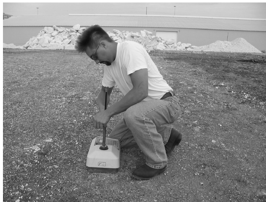
(b) Nuclear density testing on subgrade
