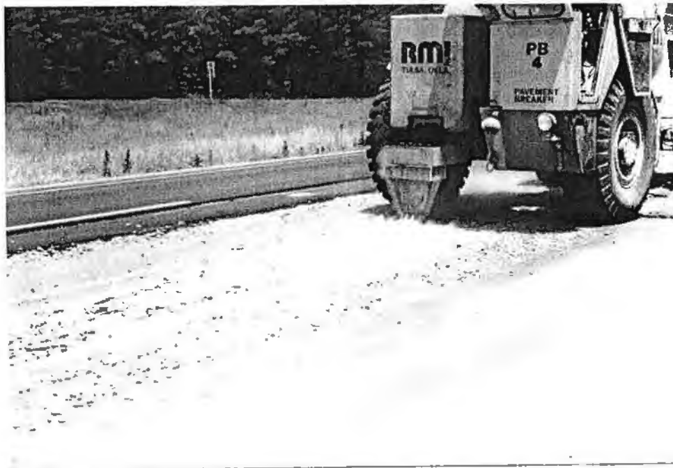
Figure 9. Rubblizing
