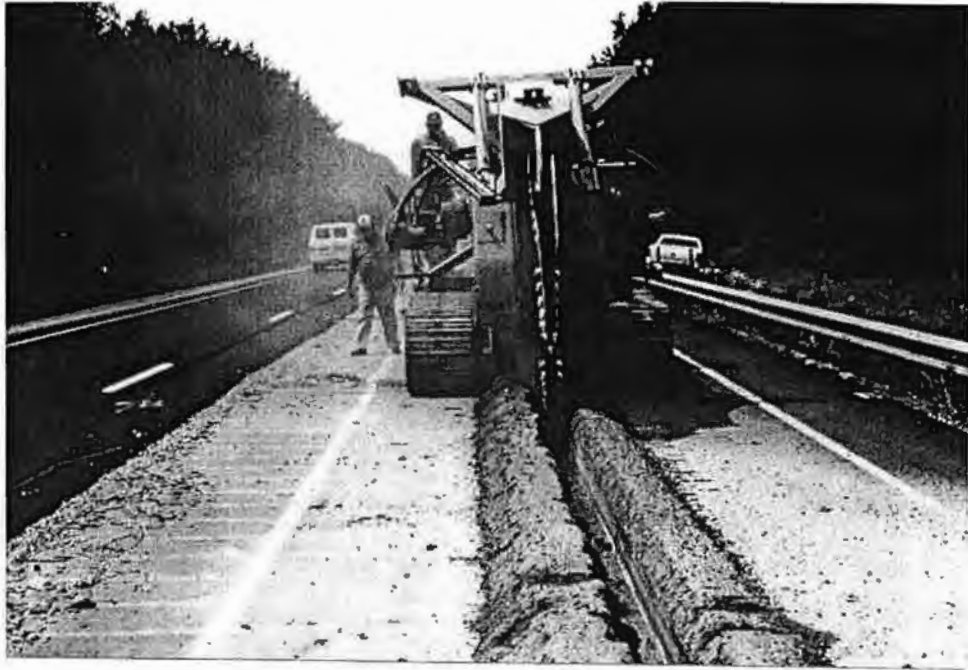
Figure 4. Trench cutting using a Ripper Saw
