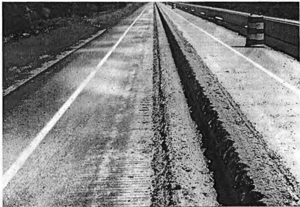
Figure 5. Trench for edge drain
