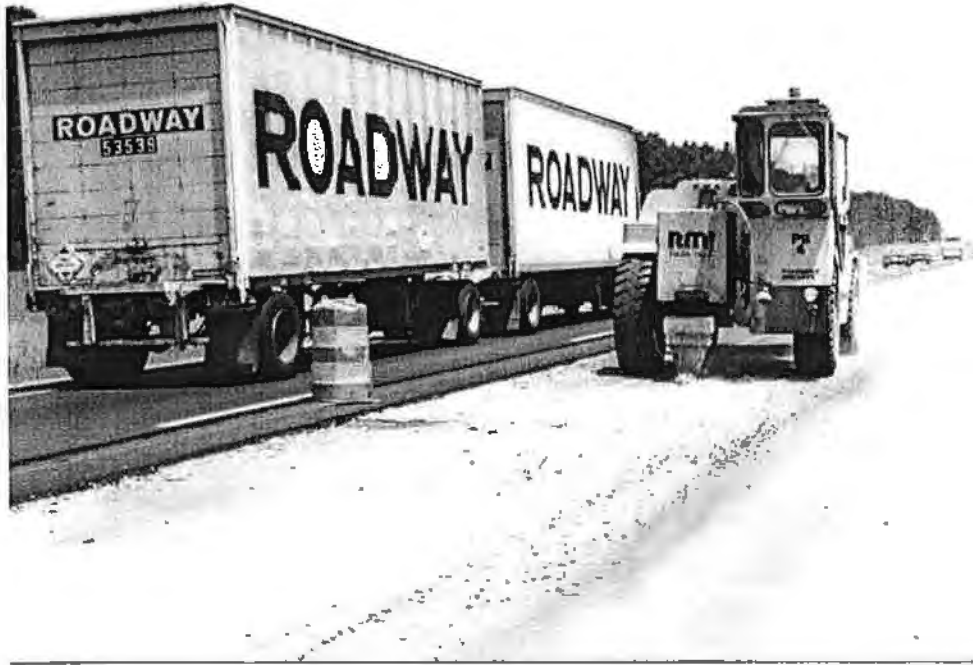
Figure 8. Rubblizing CRCP with a resonant pavement breaker
