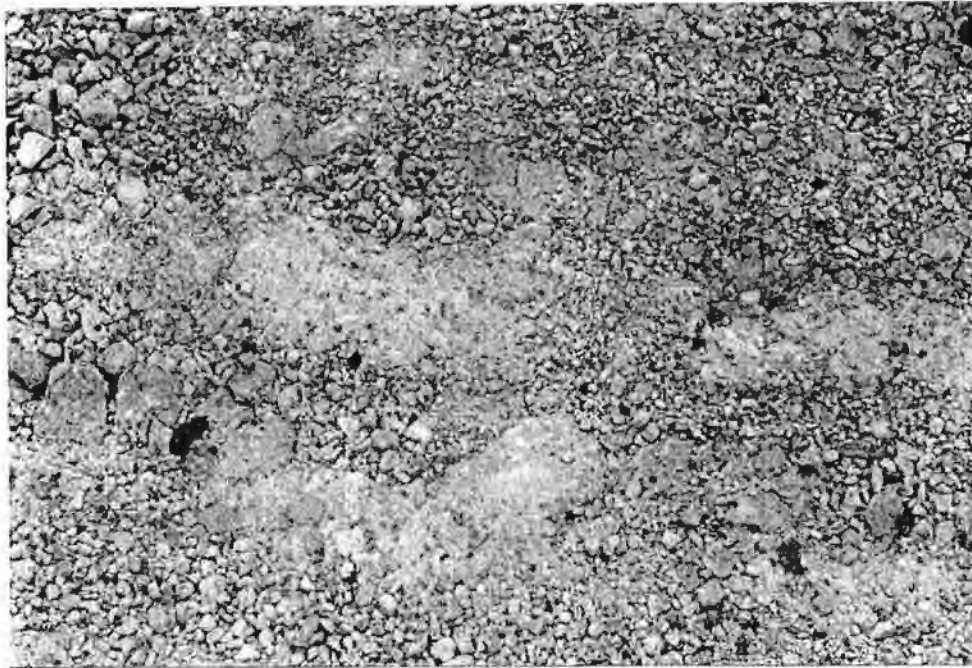
Figure 10. Rubblized continuously reinforced concrete surface
