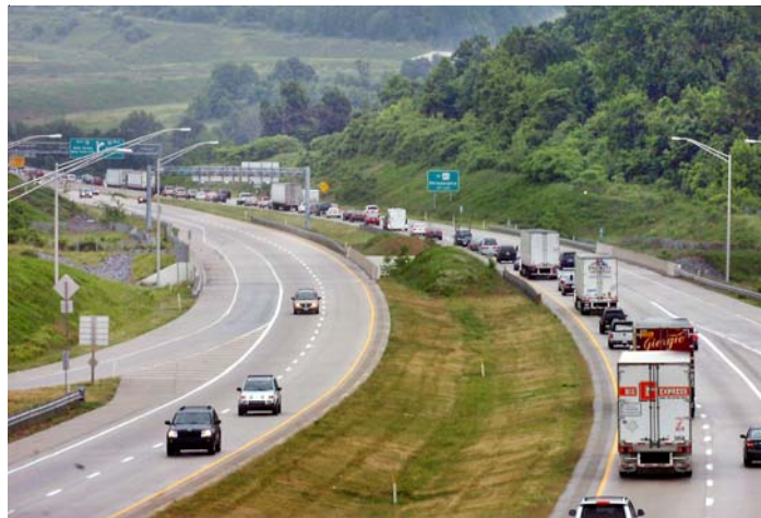
I-78 in Northampton County
