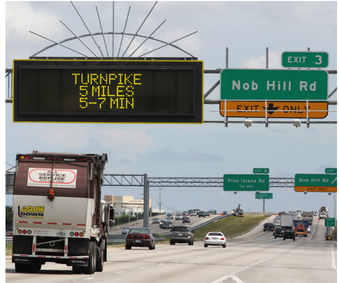
This dynamic message sign in south Florida displays the distance and approximate travel time to an important exit.
