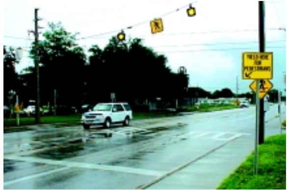
Special improvements made at the Menorah Center include the relocation of advance stop lines, a redesigned crosswalk, and the installation of overhead signals and prompting signs.
