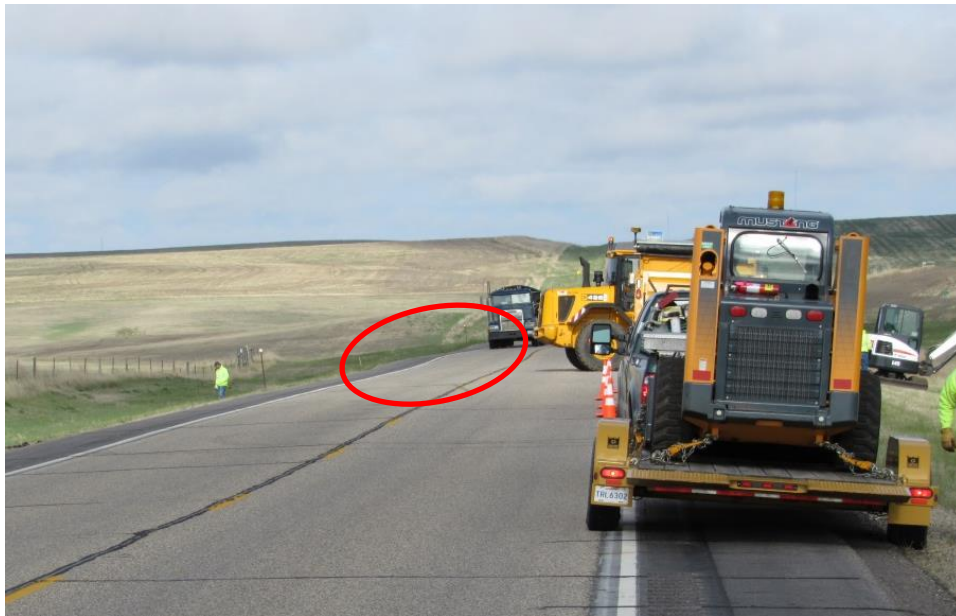
Figure 13: Site 1, settlement and/or heave in the highway near the location of the fault.
