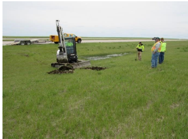
Figure 28: Site 3, soil sample location on east side of fault (heave) showing standing water on west side of fault.
