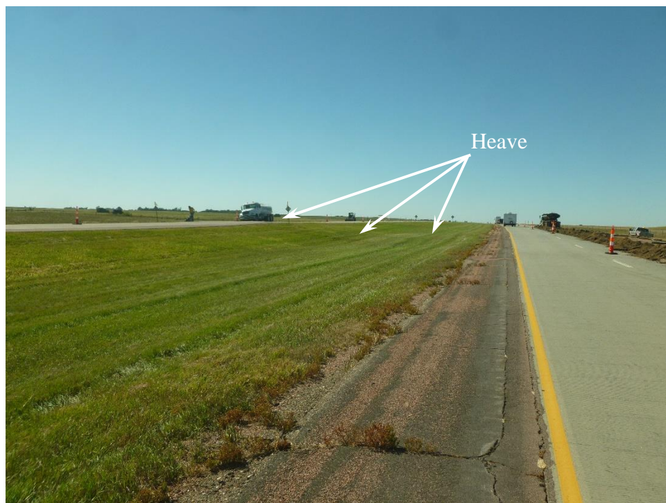
Figure 39: Site 5, heave evident across the median.
