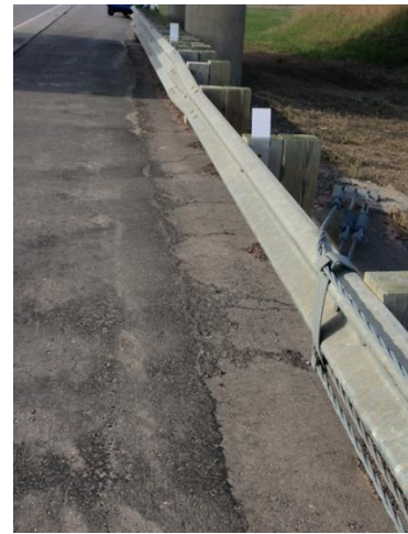
(c) Three-Strand Cable to W-Beam to Thrie Beam
