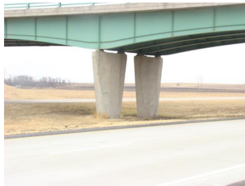
Figure 6-10: Flared Columns with No Bent Cap
