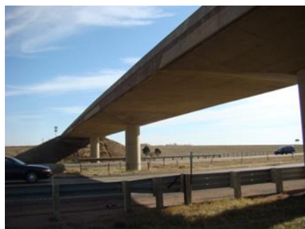
(a) Single-Circular Column Bent
