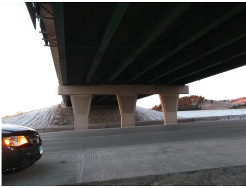
(a) Partially-Flared Columns
