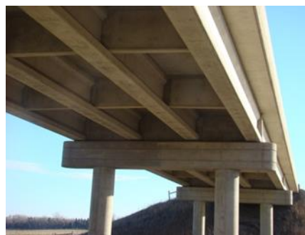
(b) Two-Circular Column Bent
