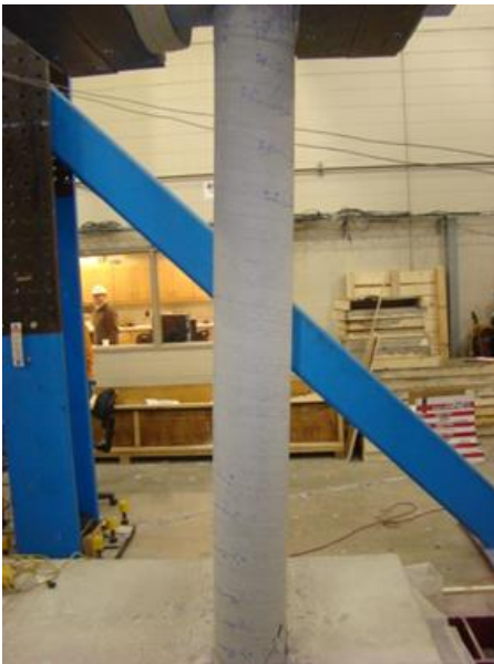
(c) Cracking in the Back Column
