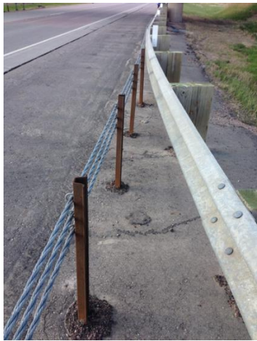
(a) Cable to W-Beam
