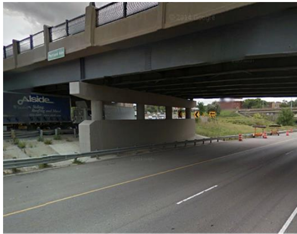
Figure 6-22: Crash Strut Retrofit (Courtesy MnDOT)
