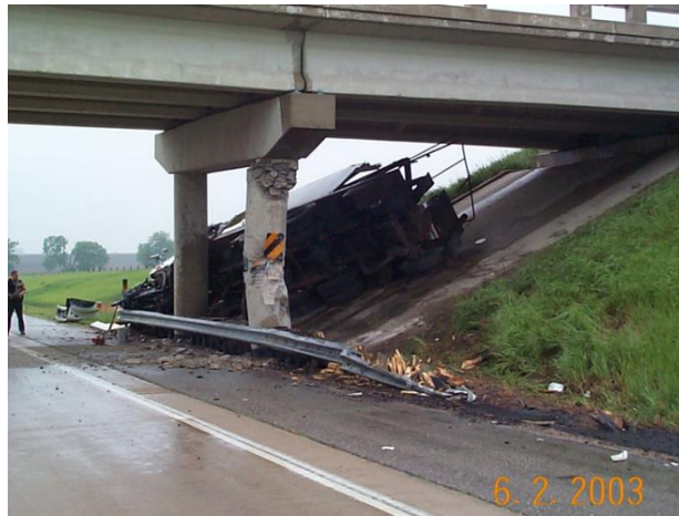
Figure 6-4: I-90 Bridge Collision near Worthington, MN (Courtesy MnDOT)
