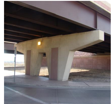
(f) Hammerhead Column
