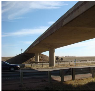
(a) Single Circular Column with Integral Cap
