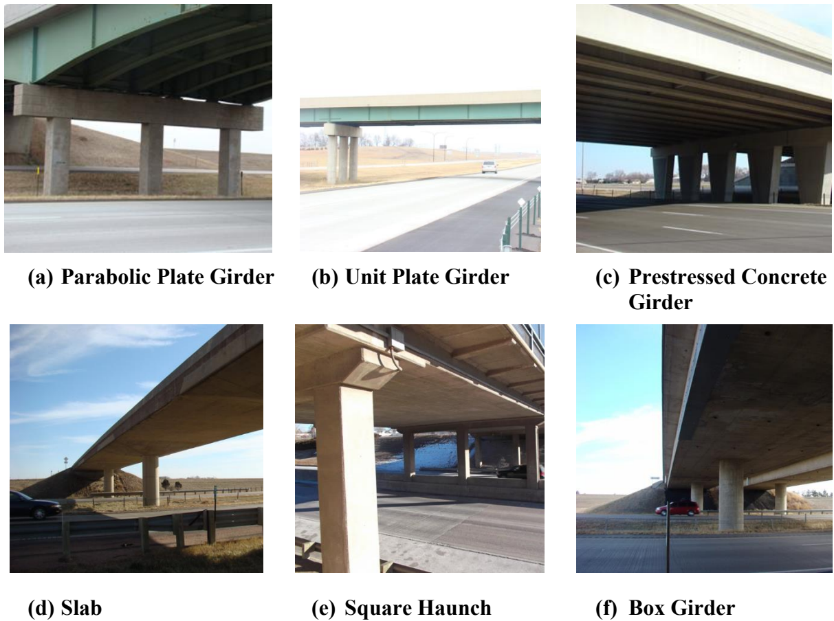
Figure 6-11: Bridge Superstructure Types
