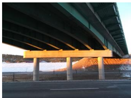
(c) Three-Circular Column Bent
