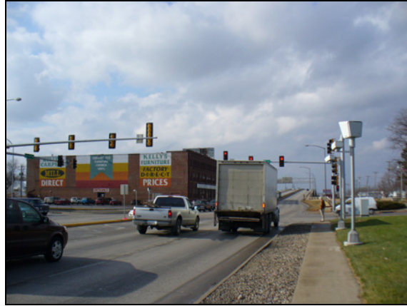
Figure 4.11. Eastbound traffic for Kanesville Blvd. and 8th St.
