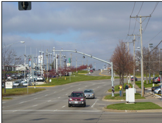
Figure 5.10. Northbound traffic for 35th St. and N. Harrison St.
