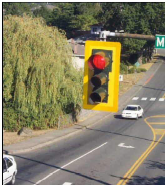
Figure 1.1. Signal with high intensity yellow retroreflective tape on backplate (Miska et al., 1998).
