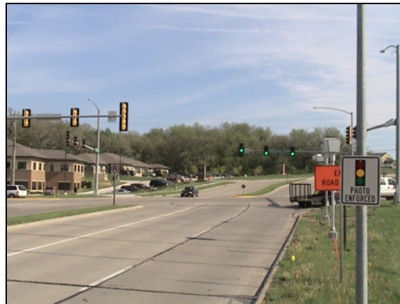
Figure 3.11. Northbound traffic for 128th St. & Hickman Rd.
