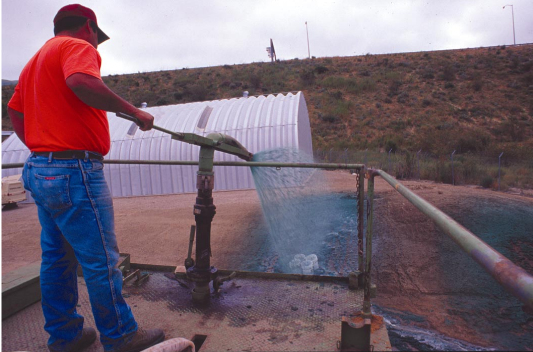
Figure 7.1. Discharging water, mulch, and mycorrhizal inoculum through a hydroseeder/mulcher.
