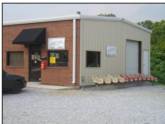
Figure 4-4. Gadsden uncovered waiting area.
