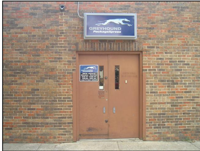
Figure 4-7. Huntsville Greyhound station package entrance.
