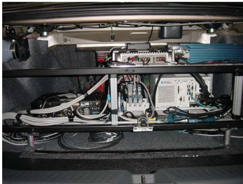
Figure 20. Trunk rack system
