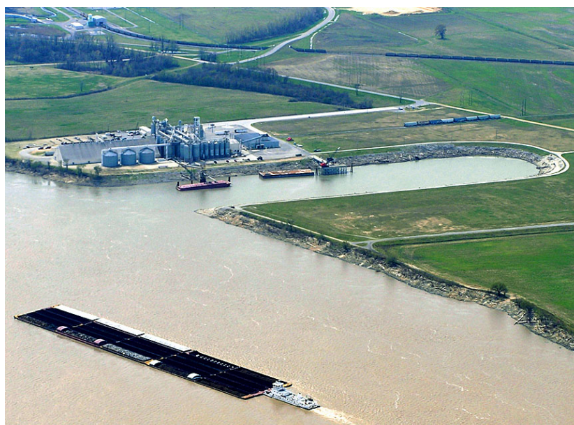
Figure 3, New Madrid County Port Authority with Barges, Trucks and Trains.
