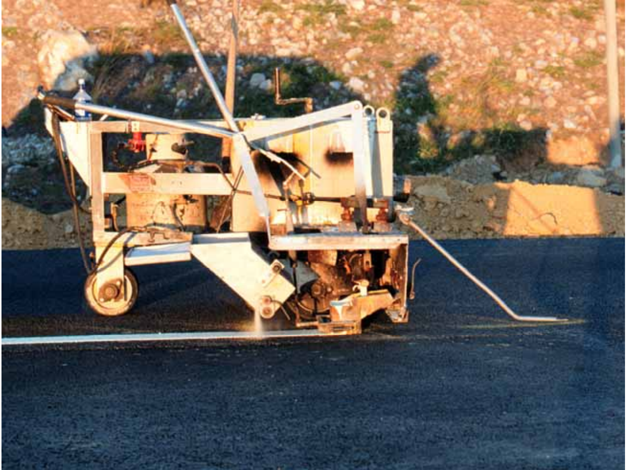
Figure 3. Photo. Application of the fluorescent thermoplastic pavement marking system.
