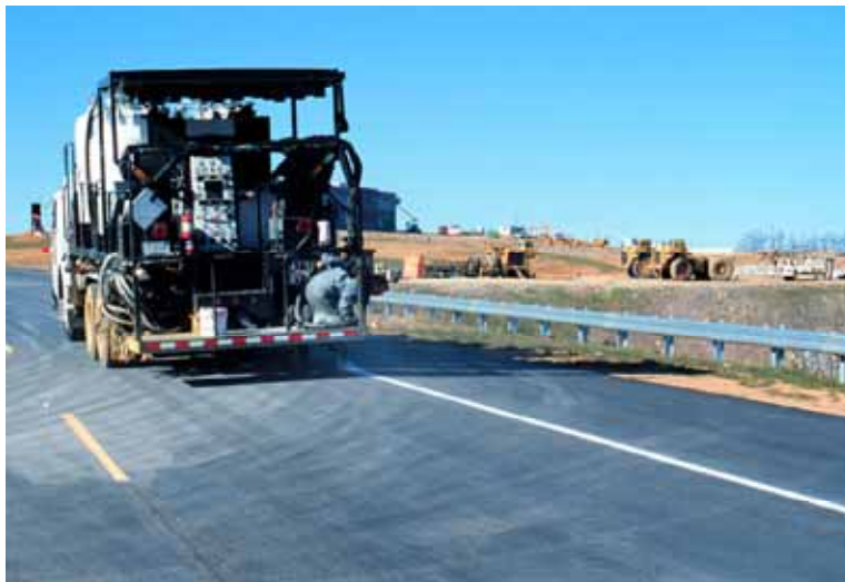
Figure 2. Photo. Application of the liquid system pavement marking.
