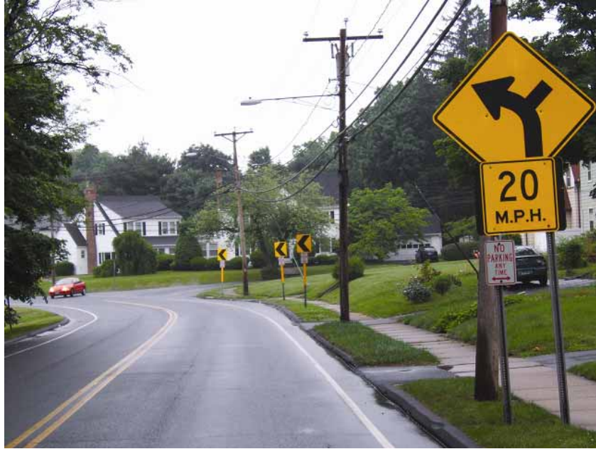
Figure 1. Photo. Example of a curve treated with enhanced delineations in Connecticut.
