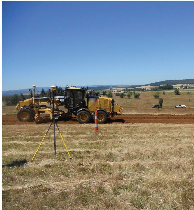
Figure 5. Photo. GNSS guided subgrade motor grader.
