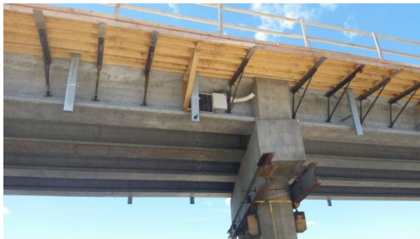
Figure 5. Data acquisition system and solar cell positioned at the intermediate bent
