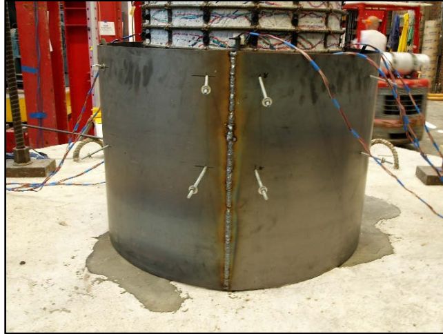
Figure 3.22: Completed butt weld on steel sleeve.
