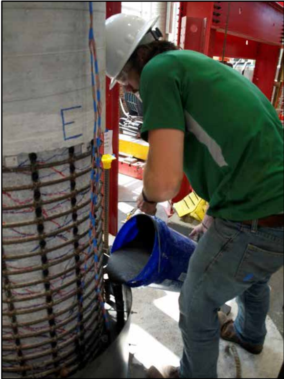
Figure 3.26: Placing grout into repair.
