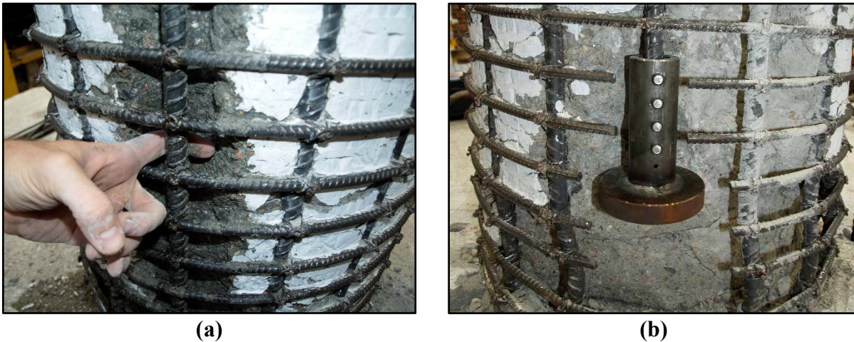
Figure 4.54: Repair #5 fractured bar anchorage mechanisms considered.
