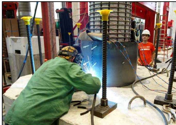
Figure 3.21: Welding the two halves of steel sleeve.
