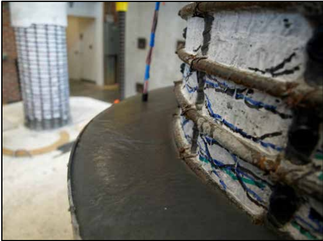
Figure 3.27: Top of repair once filled with grout.
