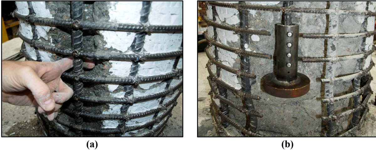
Figure 3.32: Installation of fractured bar anchorage mechanisms.
