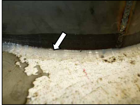
Figure 3.24: Silicone sealant at footing-steel sleeve interface.
