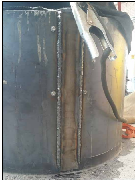
Figure 3.43: Repair #6 steel sleeve with patch of existing weld.
