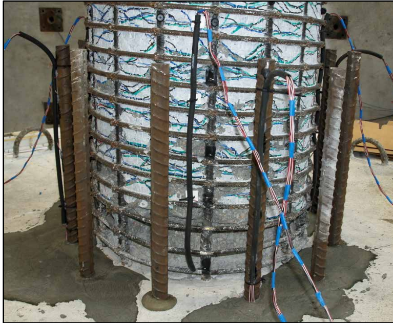
Figure 3.49: Routing of strain gage wires with rubber tubing.
