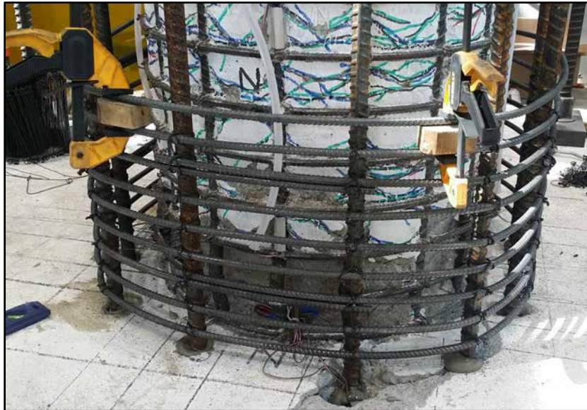
Figure 3.29: Installation of rebar hoops in Repair #4.
