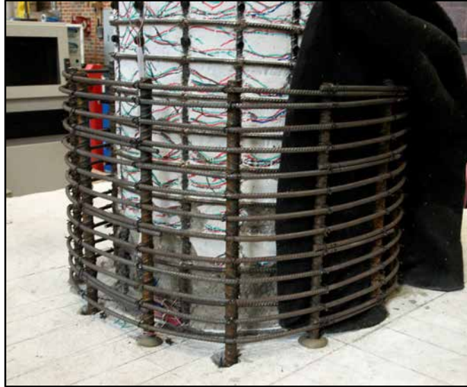
Figure 3.30: Completed rebar cage for Repair #4.
