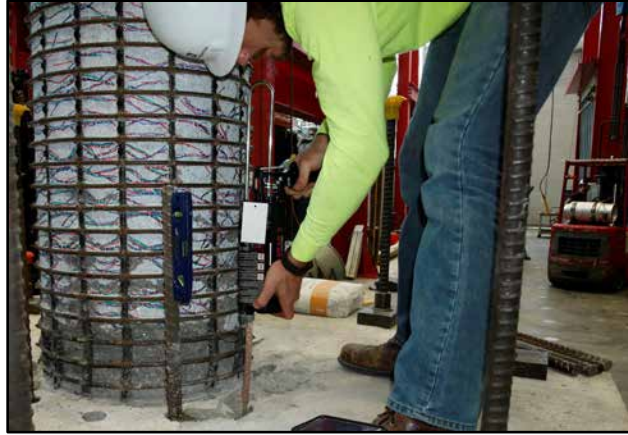
Figure 3.18: Installation of two-part epoxy into footing.
