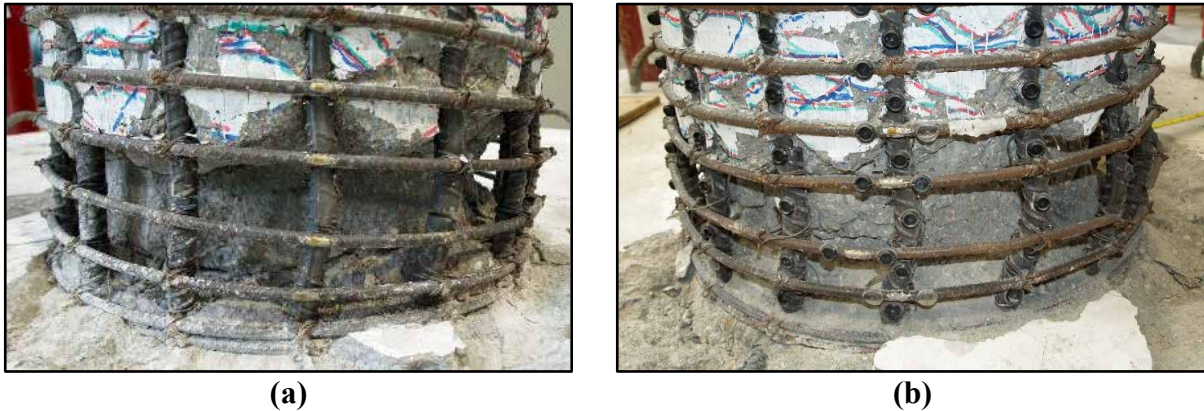
Figure 1.6: (a) Plastic hinge with buckled and fractured reinforcing bars; (b) Plastic hinge with buckled bars and fractured spiral.
