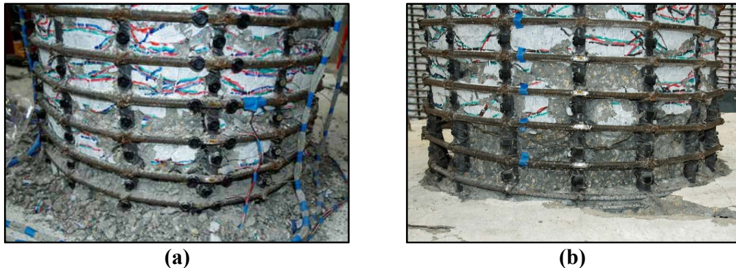
Figure 3.13: Existing plastic hinge (a) before and; (b) after crushed core removal.
