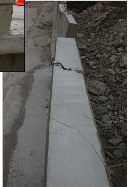
Figure 30. Bridge Rail T203 Retrofit/Repair at Location D after Test B12.
