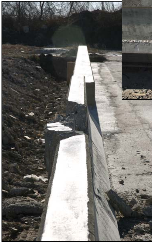
Figure 23. Bridge Rail T501 Retrofit/Repair at Location B after Test B8.
