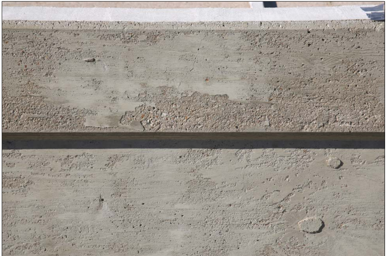
Figure 22. Bridge Rail T501 Retrofit/Repair at Location A after Test B7.
