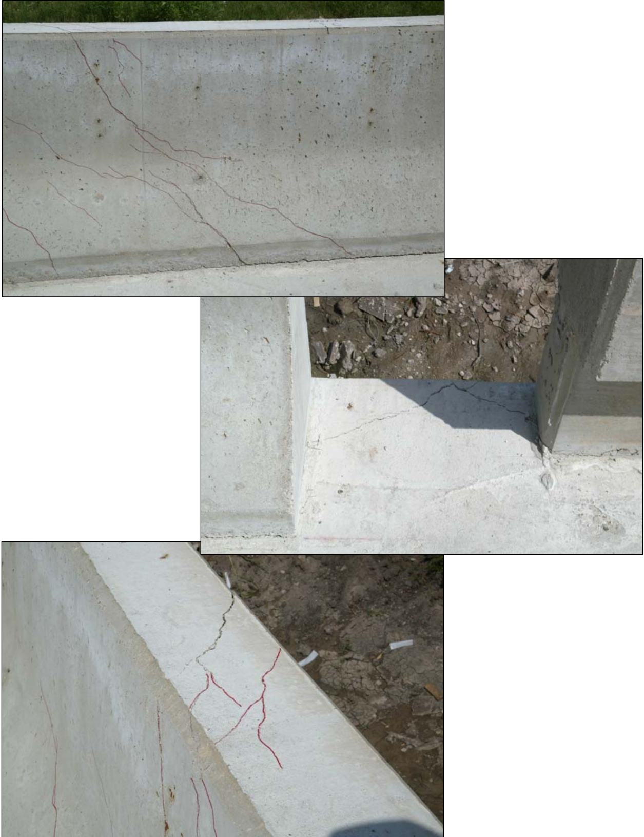
Figure 11. Bridge Rail T501 at Location C after Test S6.
