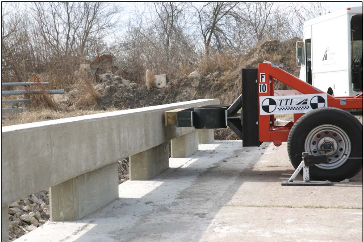
Figure 27. Retrofit/Repair for the T203 Bridge Rail before Testing.
