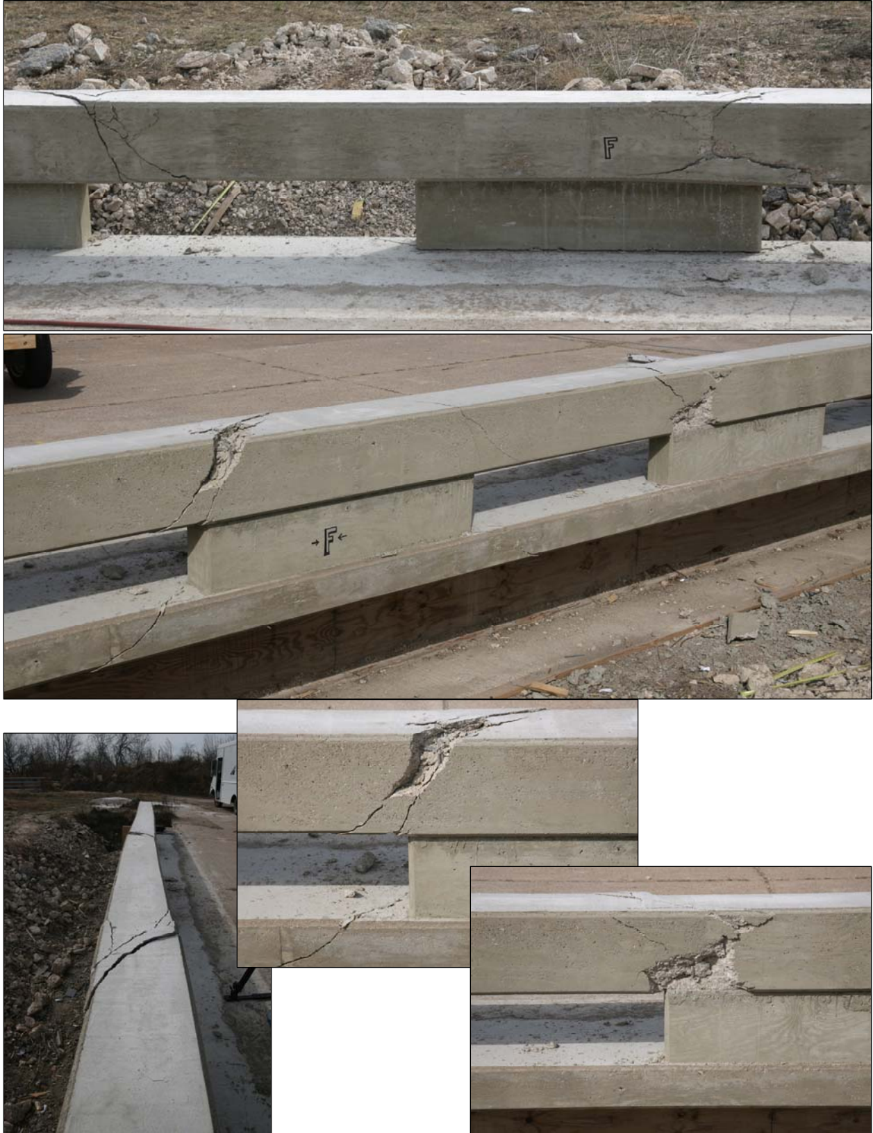
Figure 28. Bridge Rail T203 Retrofit/Repair at Location F after Test B10.
