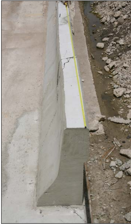
Figure 24. Bridge Rail T501 Retrofit/Repair at Location C.
