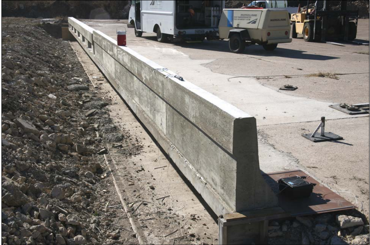
Figure 21. Retrofit/Repair for the T501 Bridge Rail before Testing.
