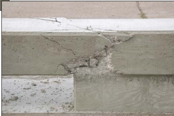
Figure 29. Bridge Rail T203 Retrofit/Repair at Location E after Test B11.
