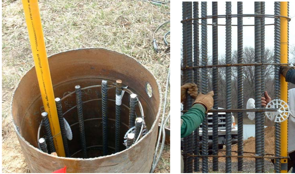
Figure 3.3: Reinforcement cage with spacers and inclinometer casing attached
