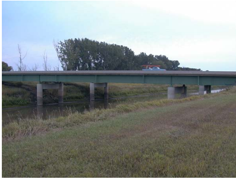
a. Photograph of bridge looking northeast.
