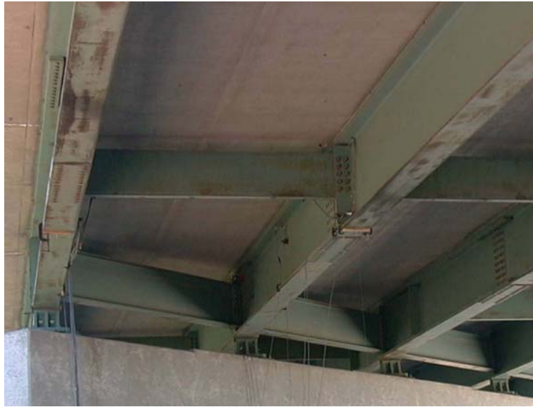
Figure 3.5. Underside view of diaphragm and girders.
