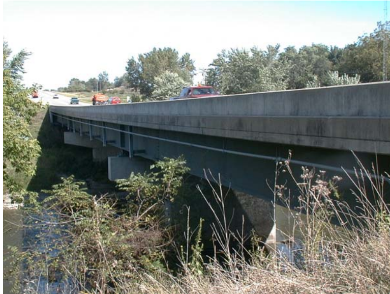
Figure 4.1. Photograph of bridge looking northeast.
