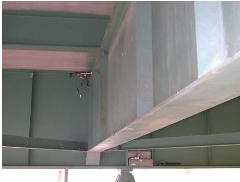
b. Photograph of floor beams and stringers under bridge deck.
