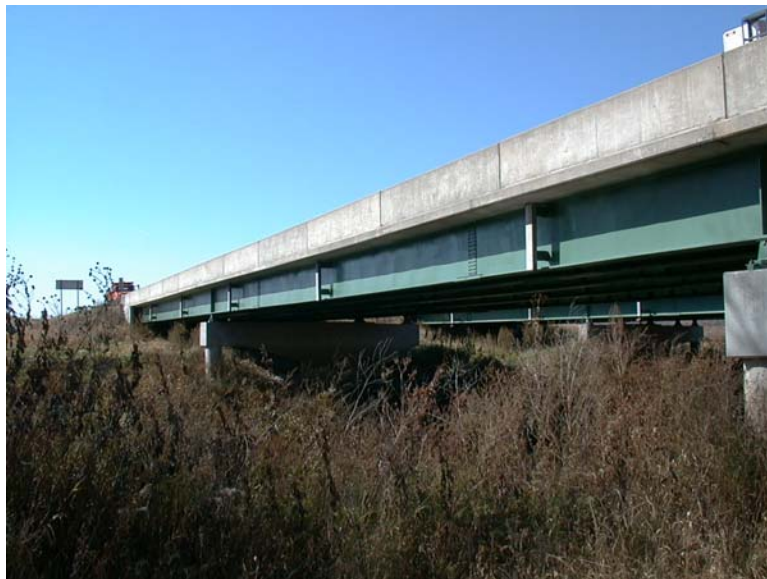
Figure 2.1. Photograph of test bridge looking northwest.
