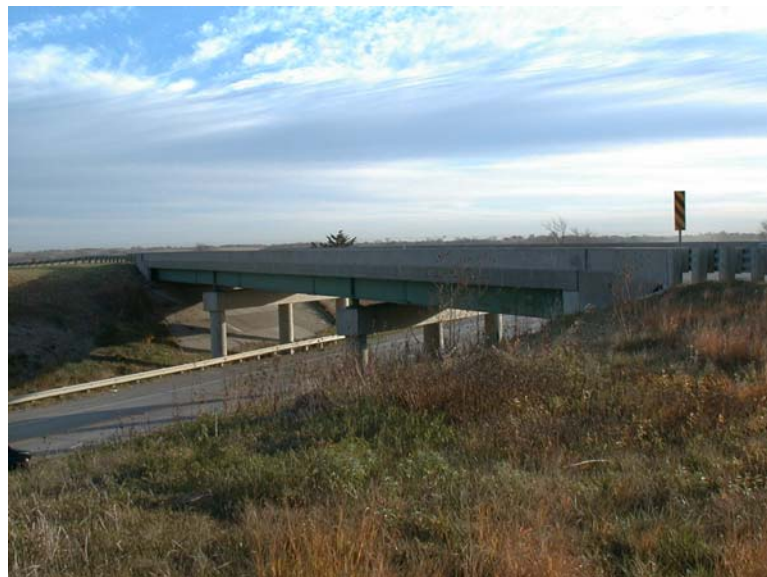
Figure 3.1. Photograph of test bridge looking northeast.
