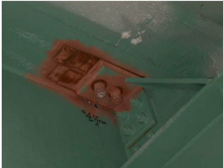
Figure 5.6. Photograph of repaired retrofit at floor beam connection.
