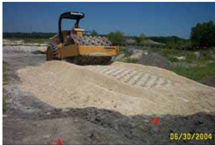
Figure 38: Compacting the test embankment
