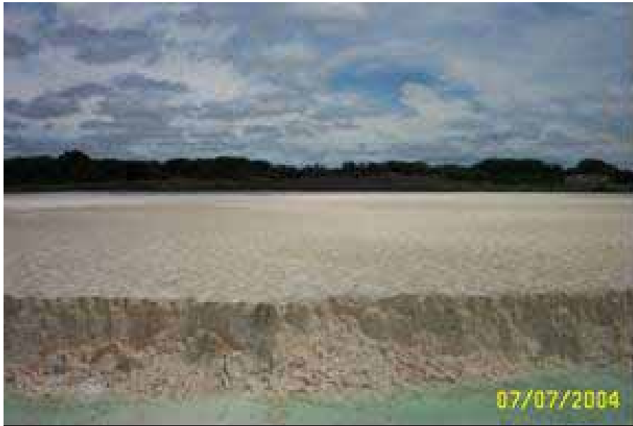
Figure 1: Lime Sludge Storage Lagoon (stockpiled)
