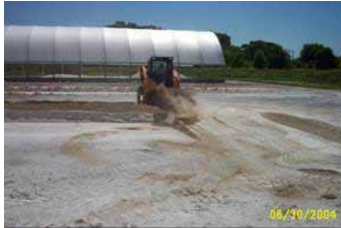
Figure 37: Mixing Lime Sludge and Fly Ash
