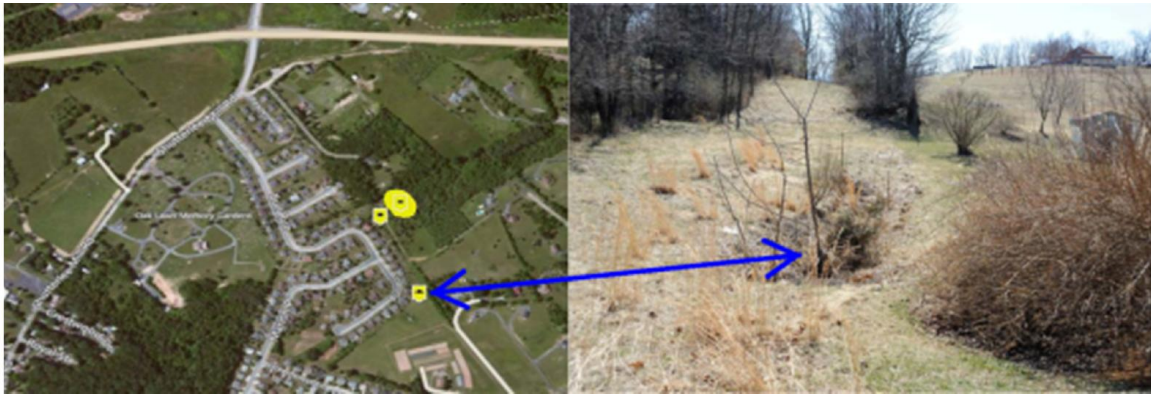
Figure 41 - Sinkhole detected in a subdivision near Staunton.
