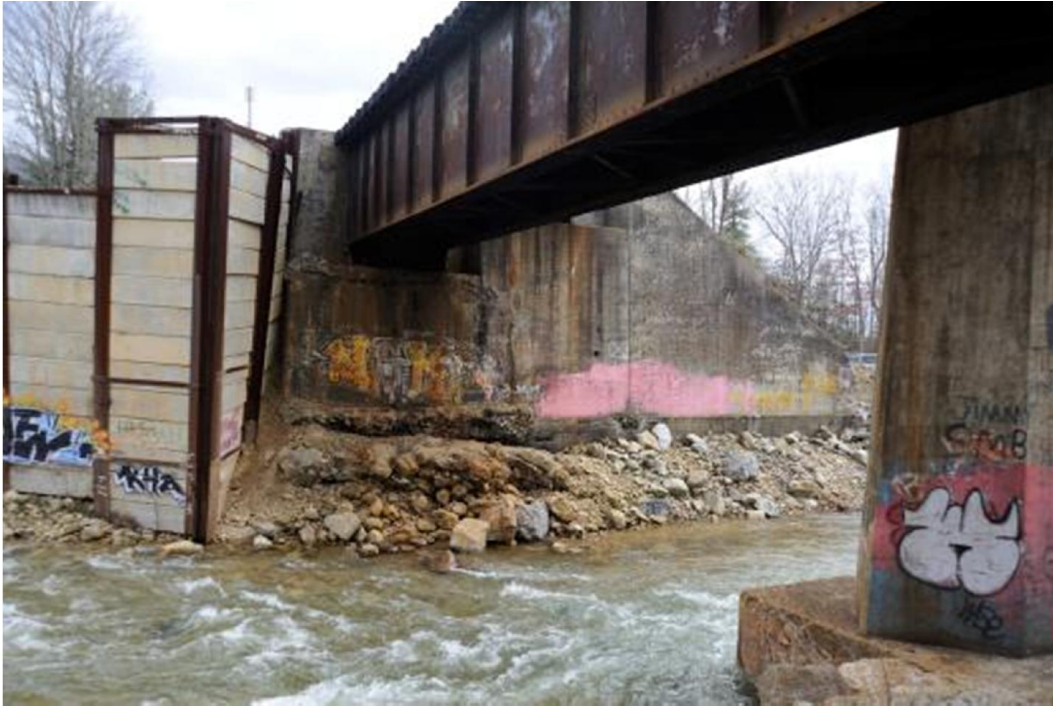
Figure 45 - Railway bridge with high InSAR displacements.
