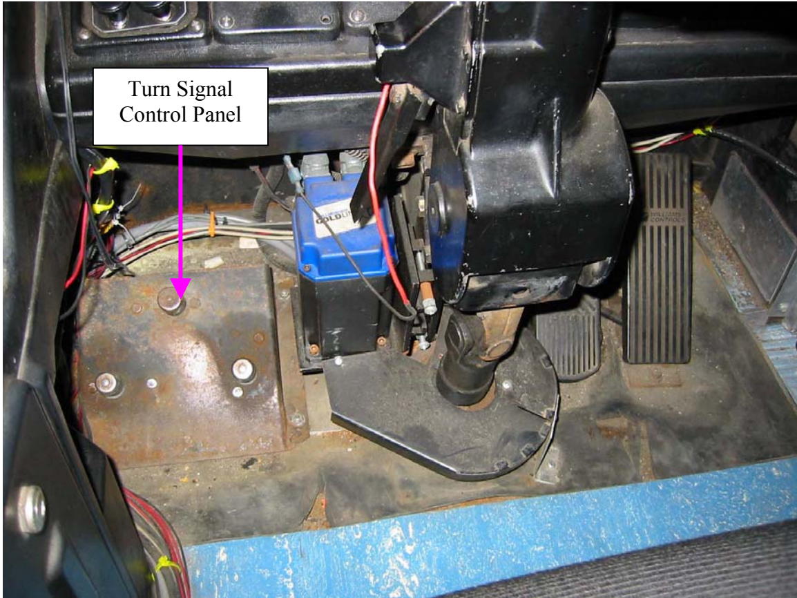
Picture 6. Technobus steering actuator. The steering servomotor is mounted to the rigid support which keeps the steering shaft in place. The steering motor is sized so as to not interfere with the drivers left foot, which is normally kept on the turn signal control panel. The steering shaft is driven by the servomotor via 3:1 Gates Polychain belt/pulley system.
