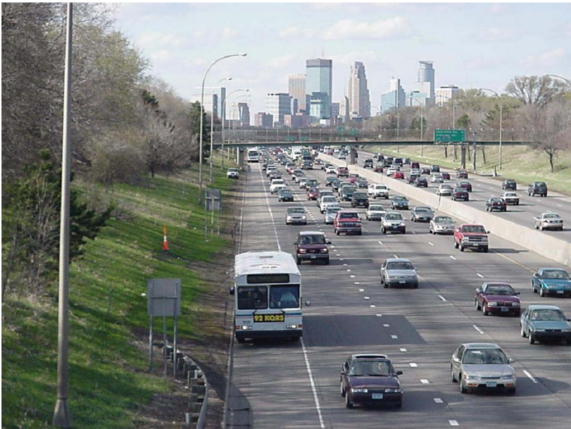
Picture 1. Illustration of a 9 ½ foot (2.9 m) wide bus operating on a 10 foot (3.05 m) wide shoulder lane. Clearly, the margin for error is significantly less for the shoulder lane than it is for normal, 12-foot (3.7 m) wide lanes.
