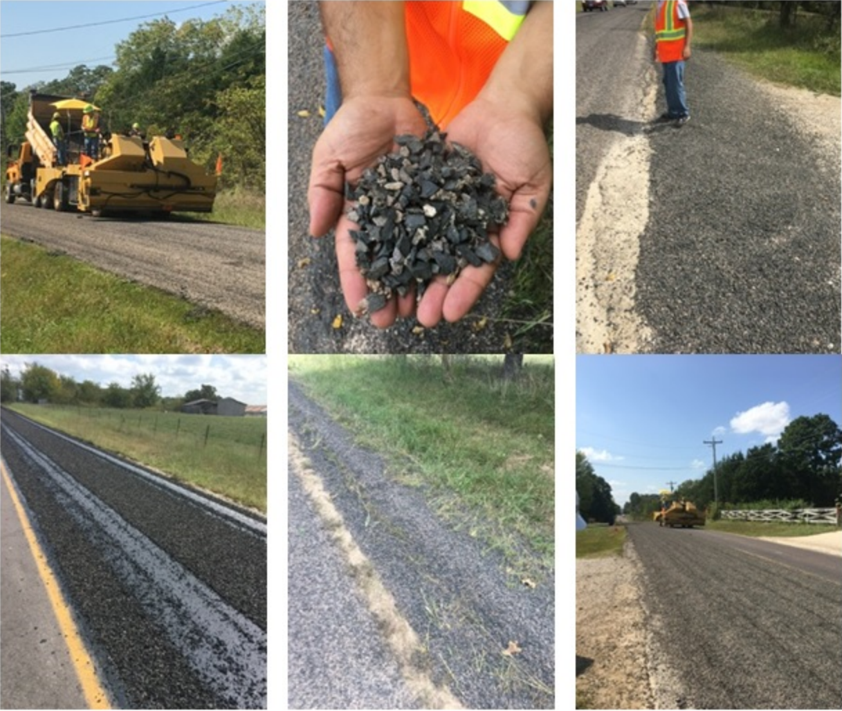
Figure C-18: Construction of field test sections
