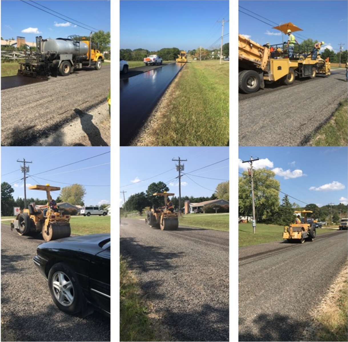
Figure C-17: Construction of field test sections
