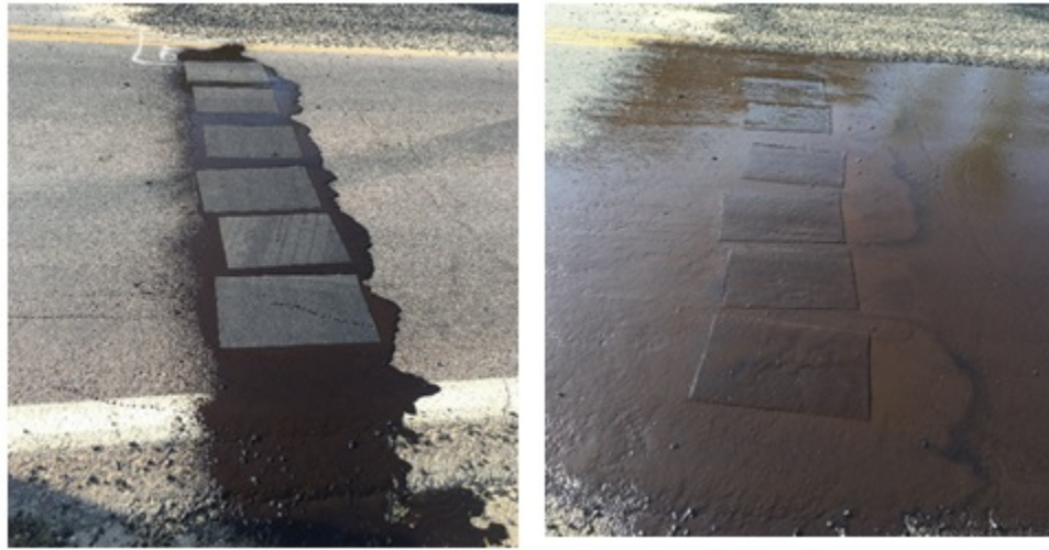
Figure 35: Collecting chip seal samples from the construction site
