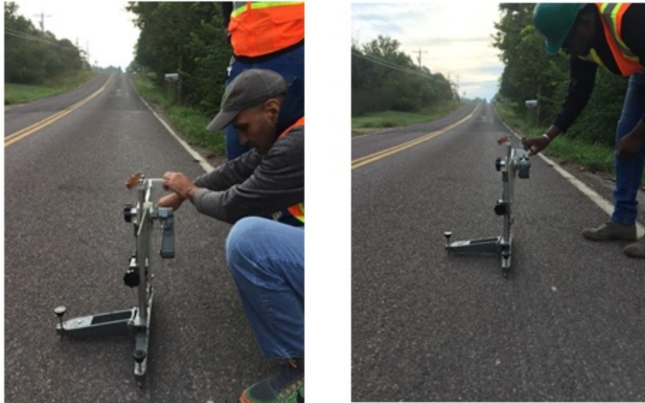
Figure 41: Field skid resistance test for a segment
