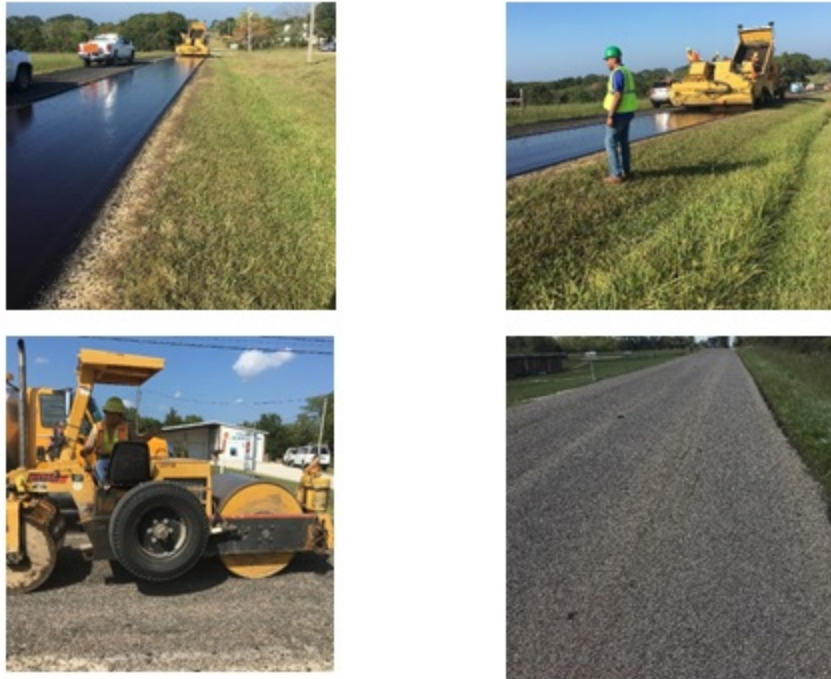
Figure 34: Construction steps of rubberized chip seal with different rubber replacement ratios
