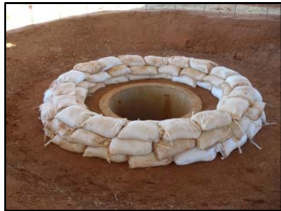
(b) sandbag inlet protection
