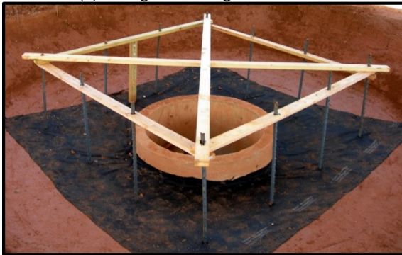
(e) T-post bracing / reinforcement
