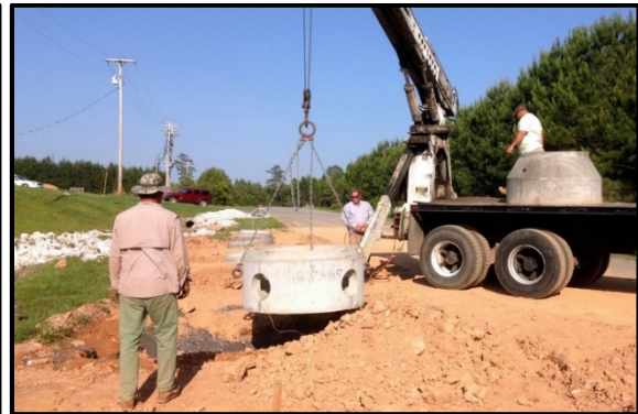
(b) installation of mock inlet structures
