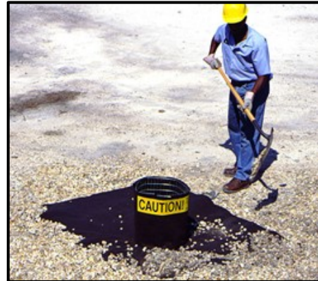
(b) grate inlet with filter fabric
