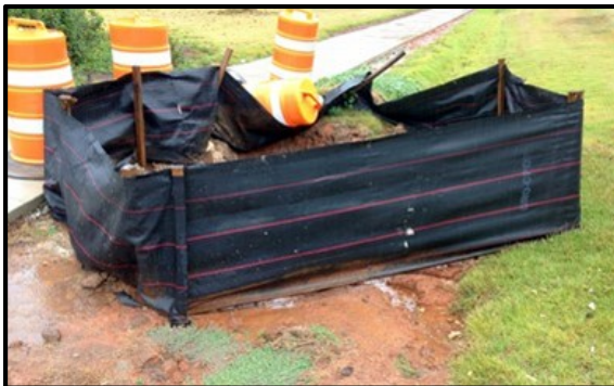
(e) improper trenching of installation
