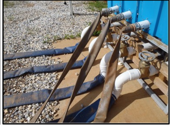
(b) inlet and outlet hoses
