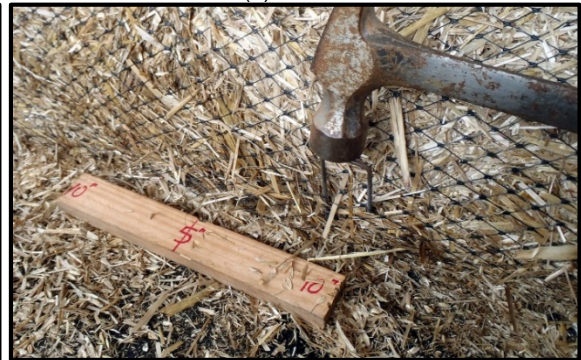
(f) MFE-I sod staple installation
