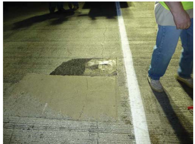
Figure D.17 Propoxy patch-III.
