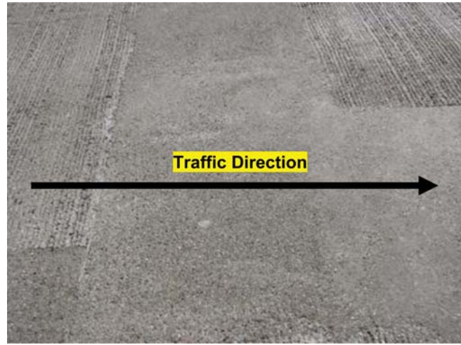
Figure B.15 Duracal AE-F patch.
