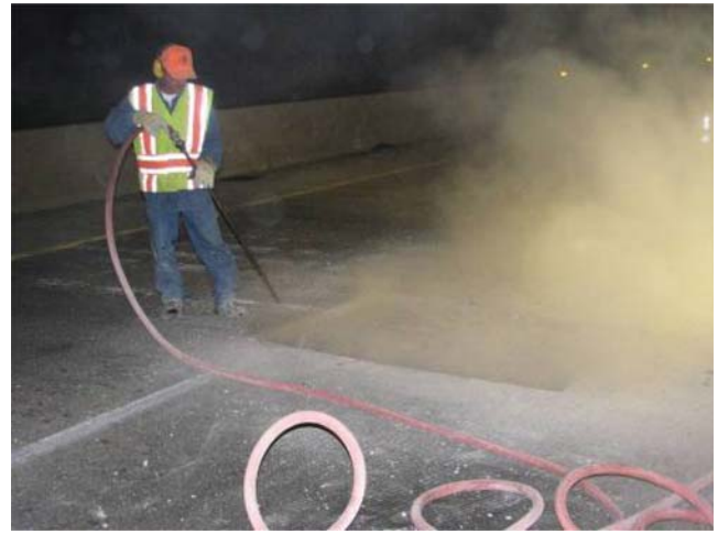
Figure 5.8 Cleaning operation.
