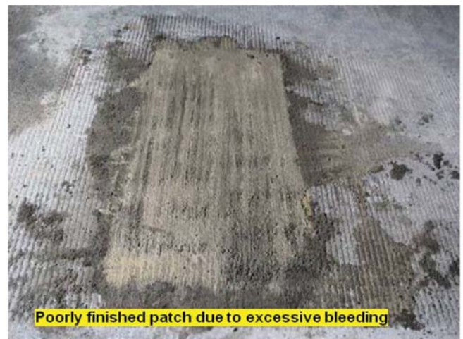
Figure 5.24 SQ-2500: finished patch-I.
