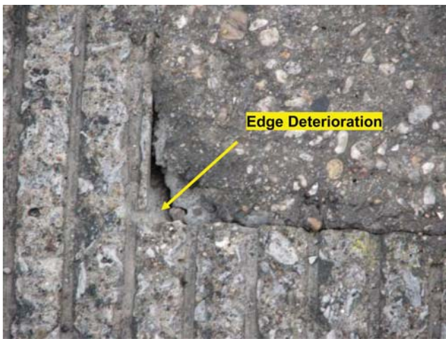
Figure A.3 HD-50 patch-I : close-up view of edge.
