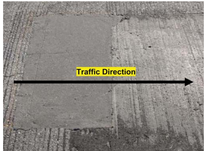
Figure B.11 SET 45 Hot Weather patch that has been replaced.
