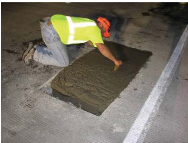
Figure 5.12 Finishing operation.
