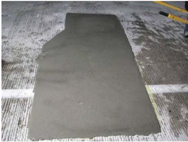
Figure 5.39 SET 45 50/50 Blend: finished patch-II.
