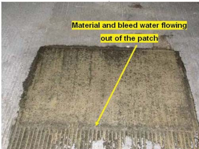
Figure 5.21 SQ-1000: finished patch.
