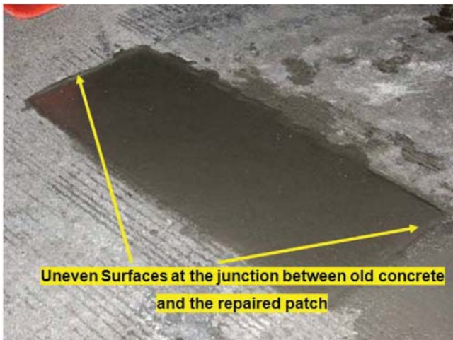
Figure 5.37 SET 45 Hot Weather: finished patch.
