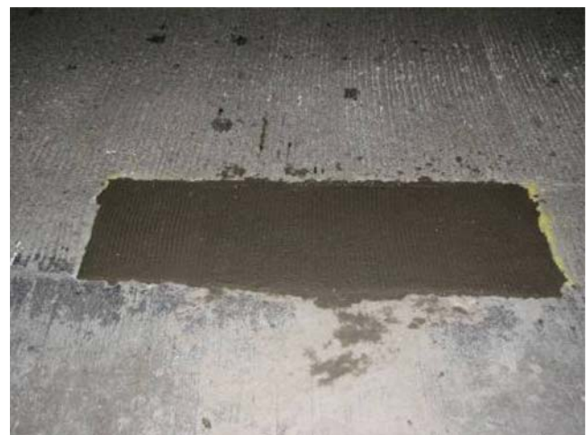
Figure 5.19 HD-50: finished patch-III.
