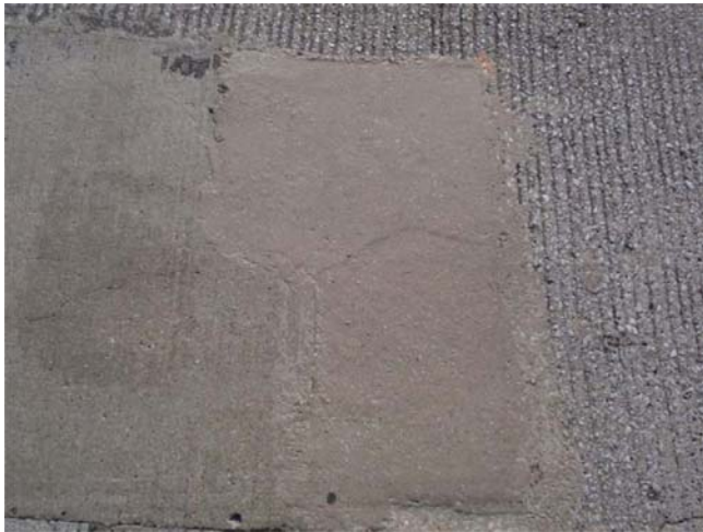
Figure C.16 Fastrak patch-III.
