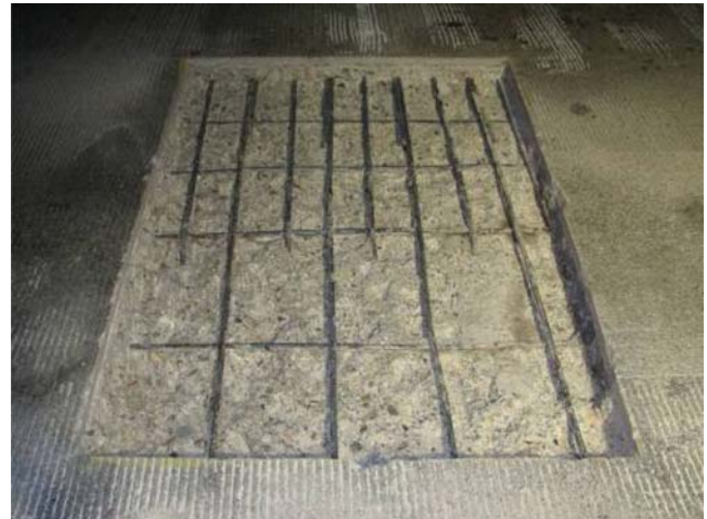
Figure 5.9 Repair area prepared for patching.
