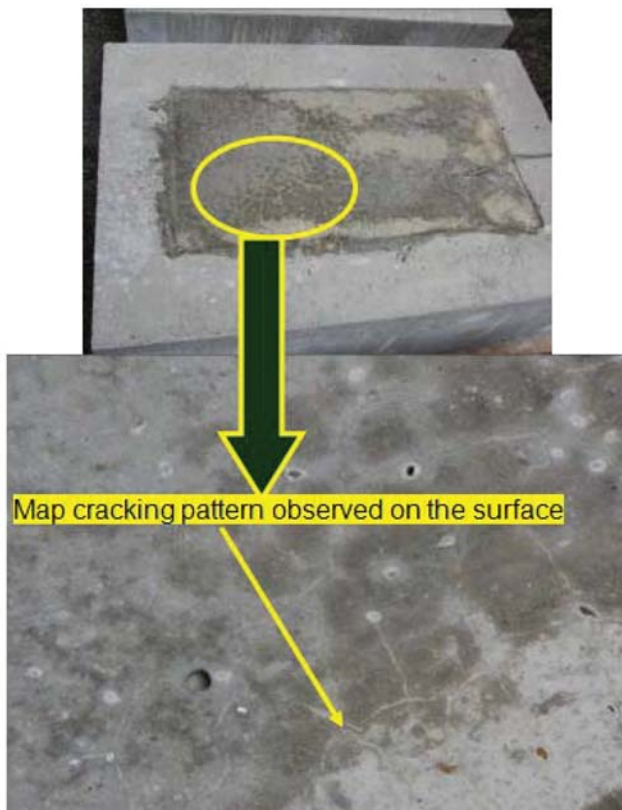
Figure 4.37 Dur-R mock-up repair—close-up view.
