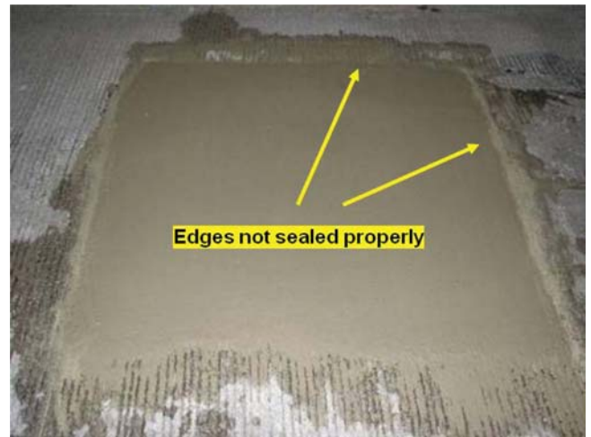
Figure 5.29 FX-928: finished patch-II.
