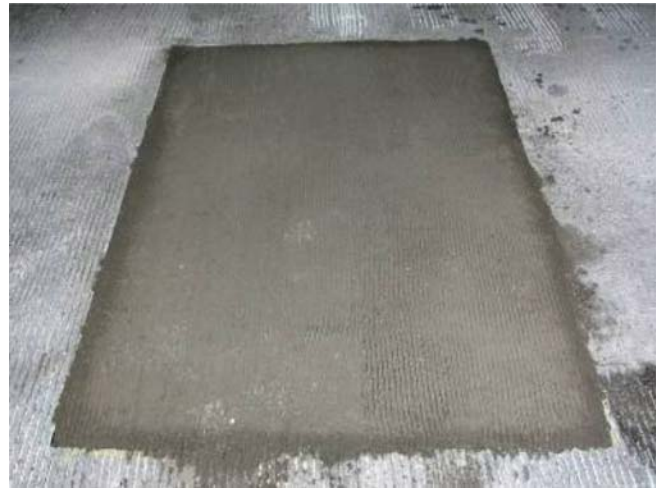
Figure 5.13 Finished patch (HD).
