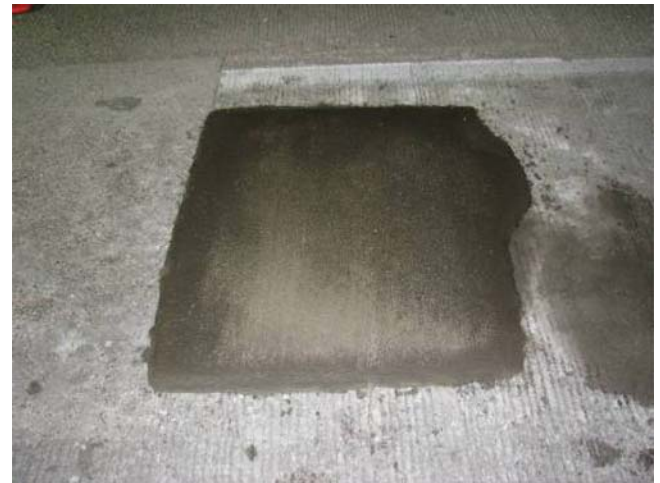
Figure 5.38 SET 45 50/50 Blend: finished patch-I.
