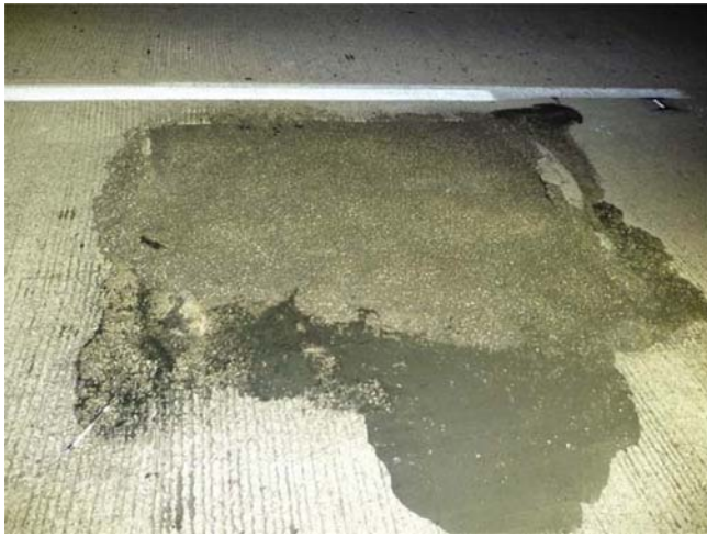
Figure D.14 Asphalt concrete in place of Zero C materials.
