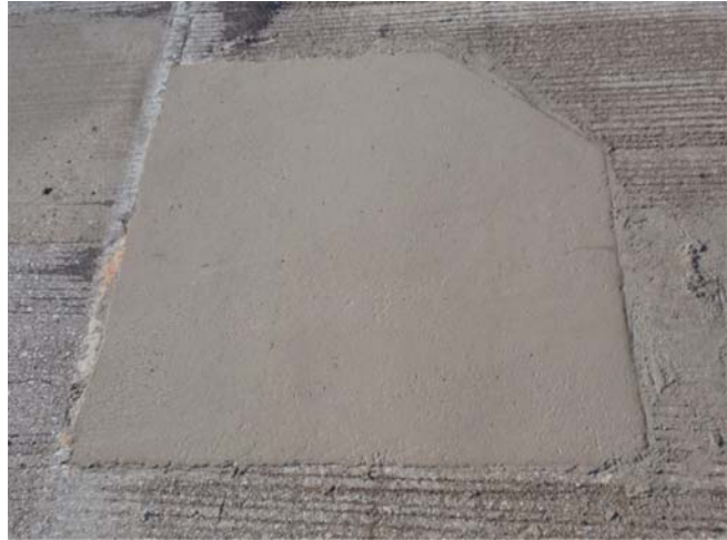
Figure C.14 Fastrak patch-I.
