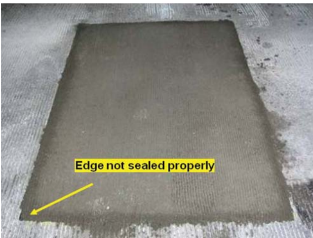
Figure 5.17 HD-50: finished patch-I.
