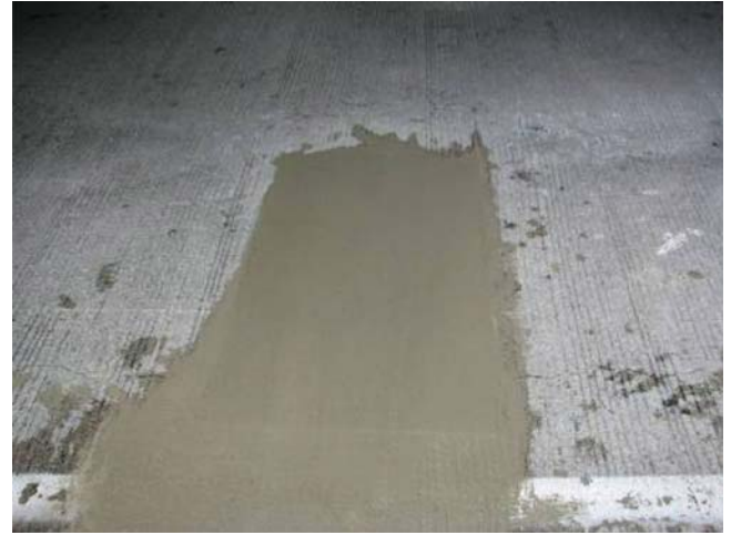
Figure 5.28 FX-928: finished patch-I.
