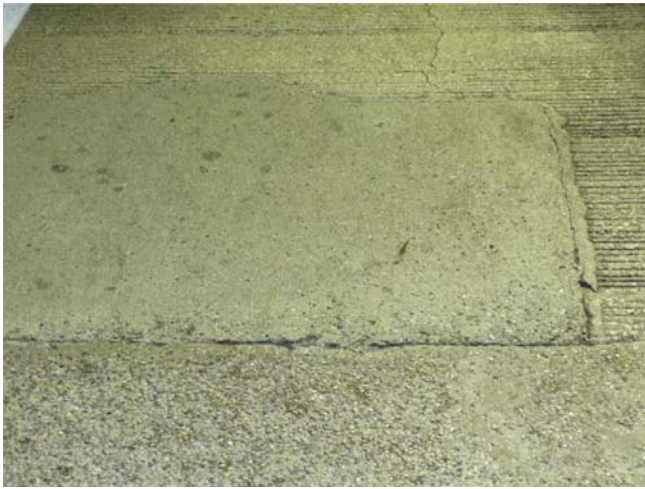
Figure D.9 SET 45 R patch area.
