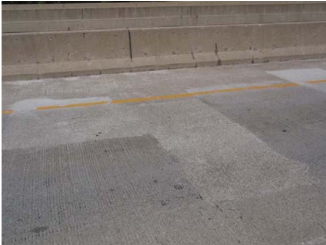
Figure C.12 Duracal AE Additional patches inspection.
