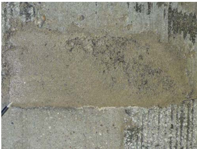
Figure D.15 Propoxy 2500 patch-I.
