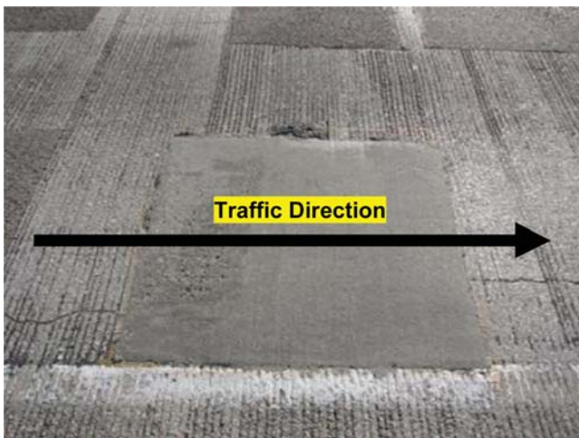
Figure B.10 SET 45 Regular patch that has been replaced.
