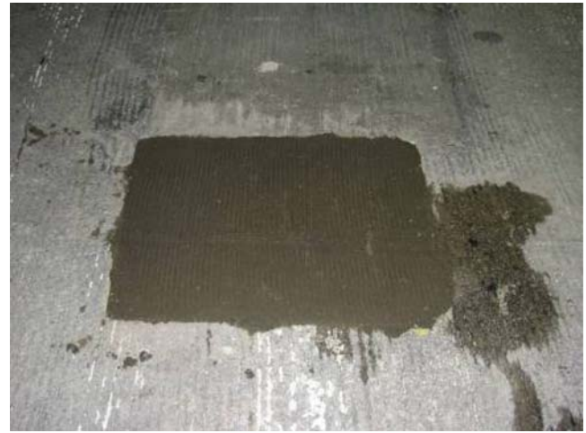
Figure 5.18 HD-50: finished patch-II.
