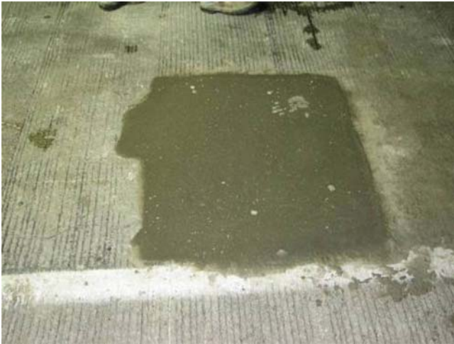
Figure 5.36 SET 45 Regular: finished patch.
