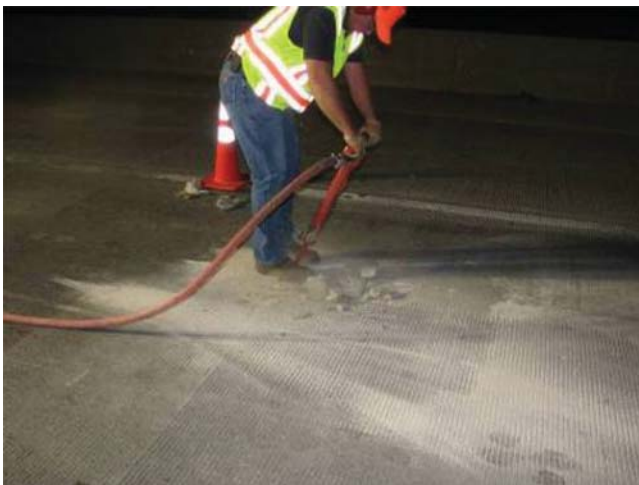
Figure 5.7 Jackhammering operation.
