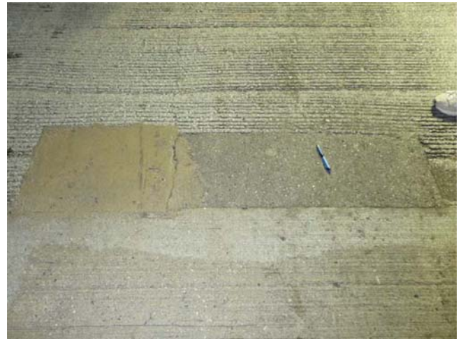
Figure D.16 Propoxy 2500 patch-II.
