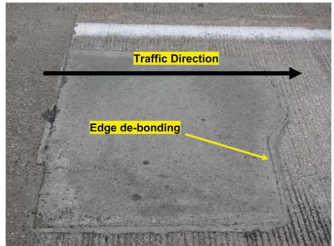
Figure A.15 SET 45 50/50 Blend patch-I.
