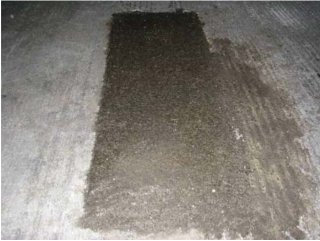
Figure 5.25 SQ-2500: finished patch-II.
