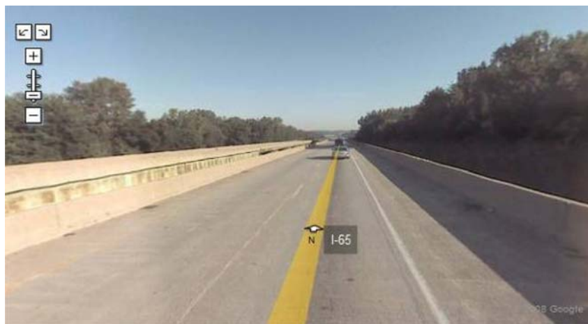
Figure 5.2 View of the bridge deck on I-65 NB. (Courtesy: Google Maps.)
