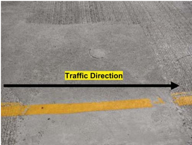
Figure B.14 Duracal AE patch.
