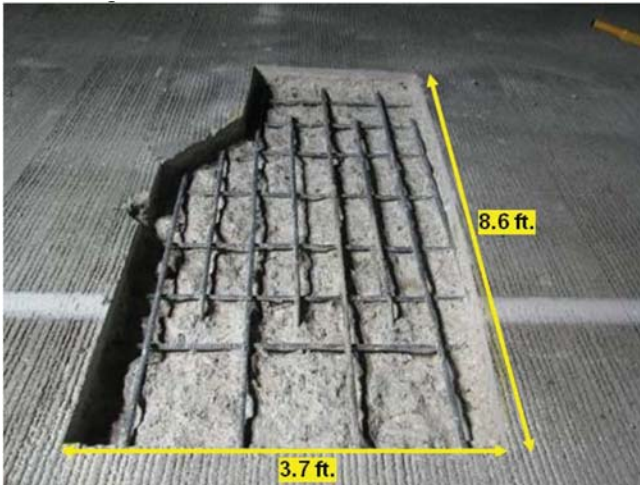
Figure 5.35 SET 45 50/50 Blend: patch area-II.
