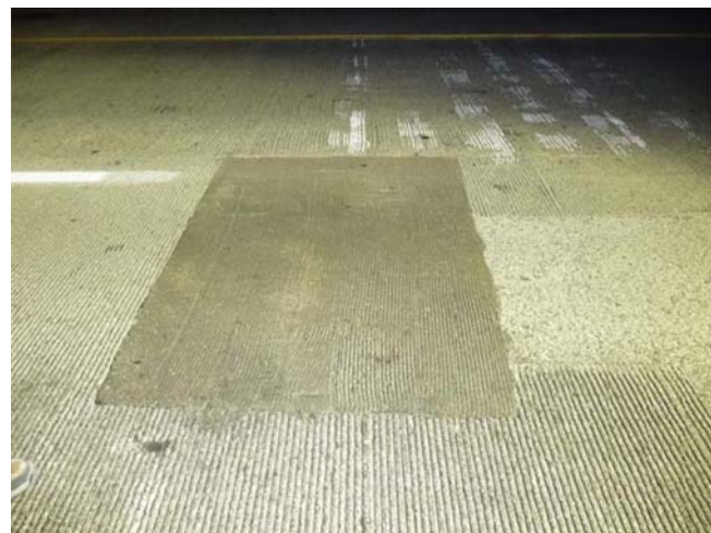
Figure D.1 HD-50 patch-I.
