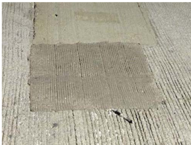
Figure D.2 HD-50 patch-II.
