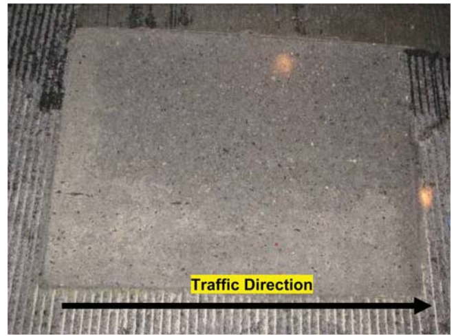
Figure A.6 SikaQuick-1000 patch condition two days
