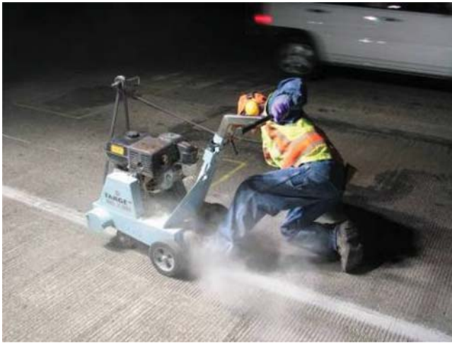
Figure 5.6 Saw-cutting operation.
