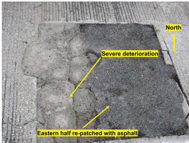
Figure A.13 SET 45 Regular patch.
