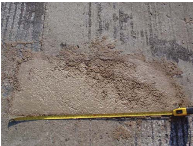
Figure C.17 Pro-Poxy 2500 patch-I.
