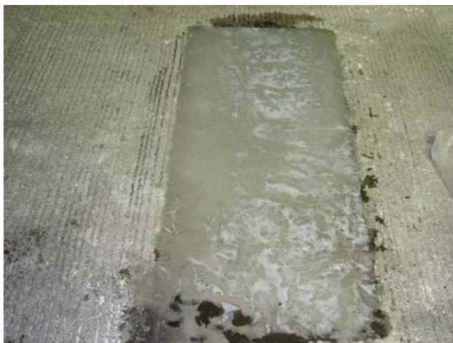
Figure 5.31 ThoRoc 10-60 finished patch.
