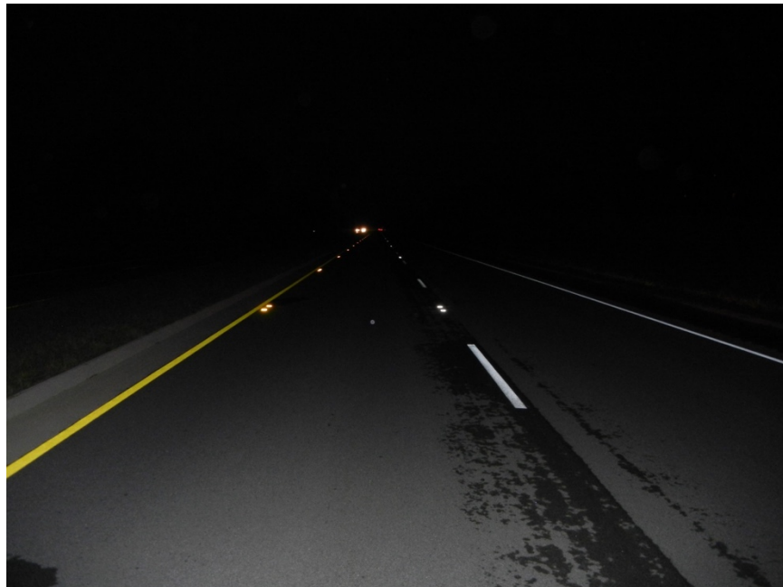
Jessamine County; US 27; Recessed Marker; Pavement Damp
