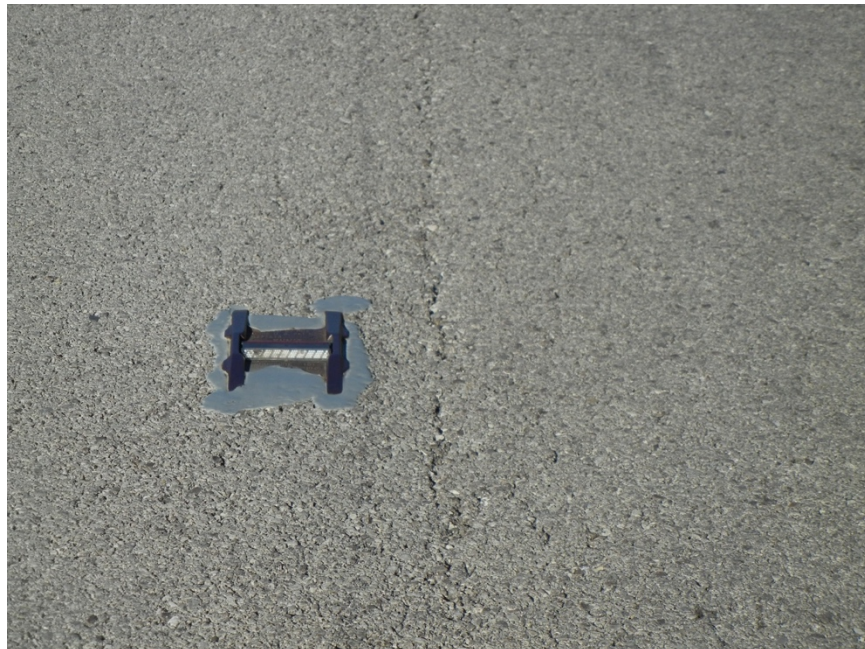
Type V Snowplowable Marker; Installed Few Inches from Pavement Joint
