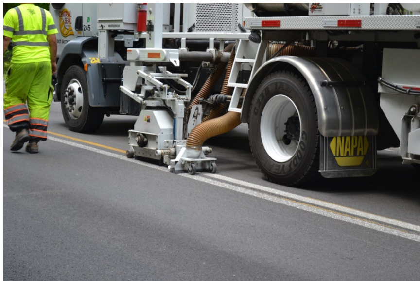
Groove Cut for Recessed Wet-Reflective Paint
