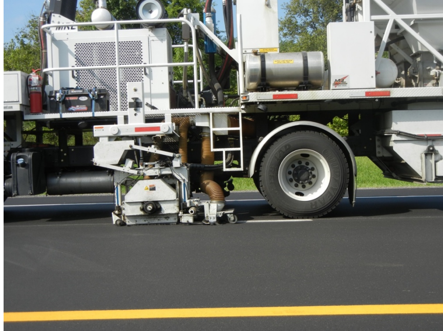
Installation of Recessed Marker
