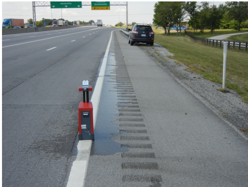
Simpson County; I-65; Spray Thermoplastic; Wet Data Collection
