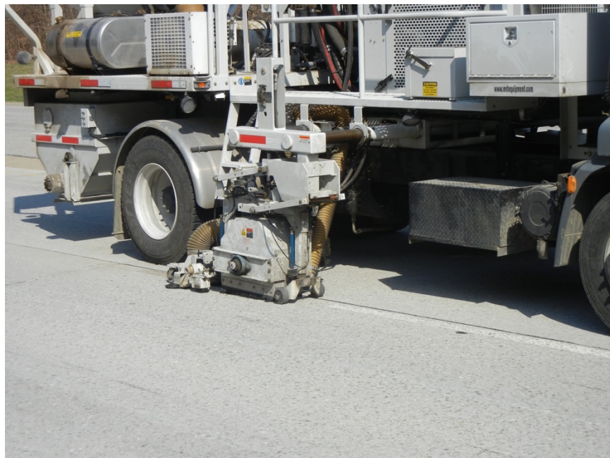
Recessed Marker Installation; Concrete Pavement
