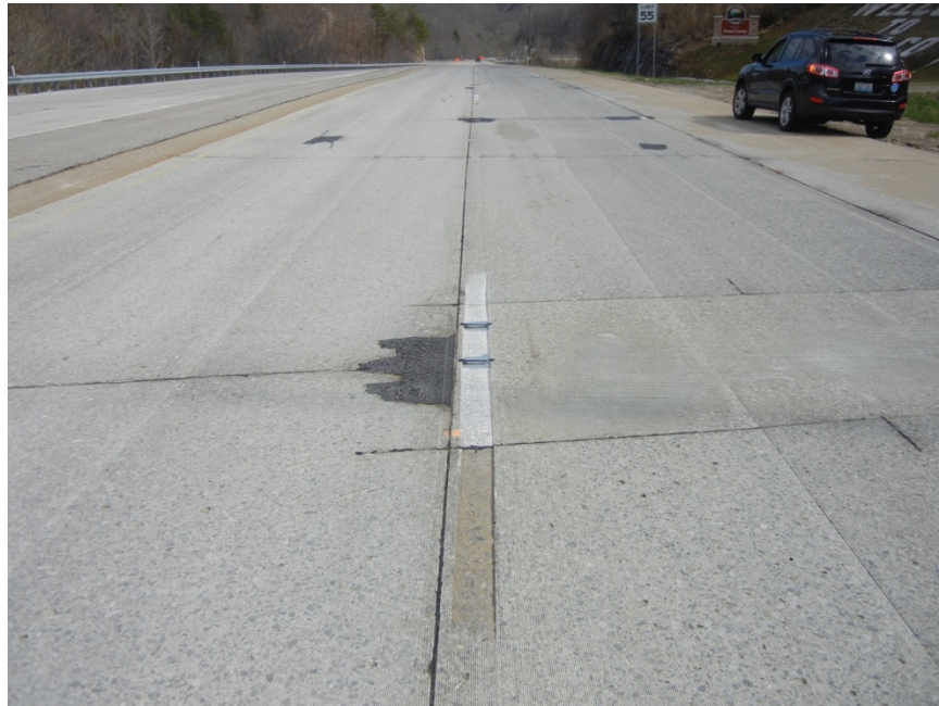
Comparison New and Old Recessed Marker Groove
