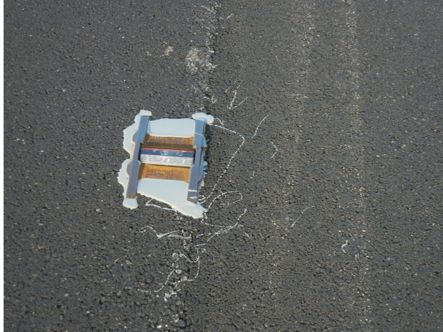
Type V Snowplowable marker; Installed at Pavement Joint
