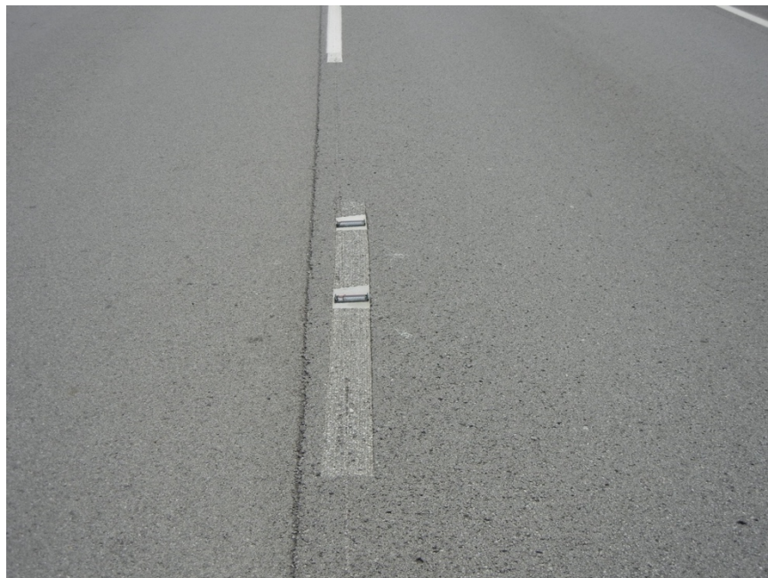
Recessed marker; Original Design
