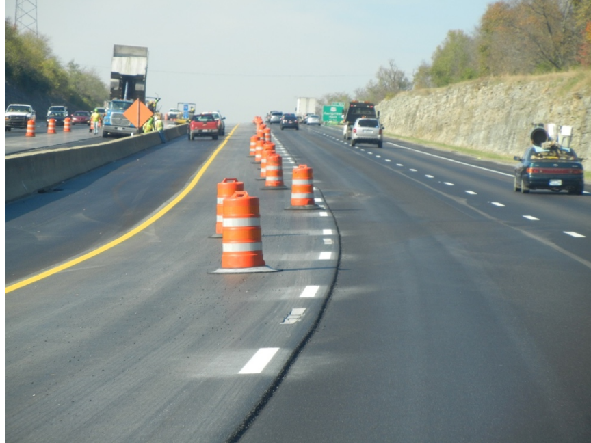
Recessed Marker Installed off Pavement Joint
