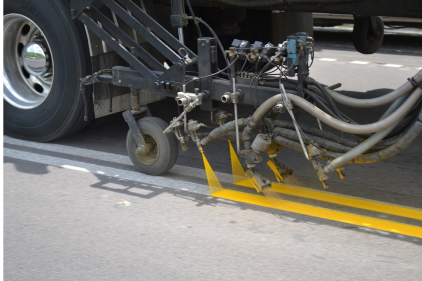
Install Recessed Wet-Reflective Paint
