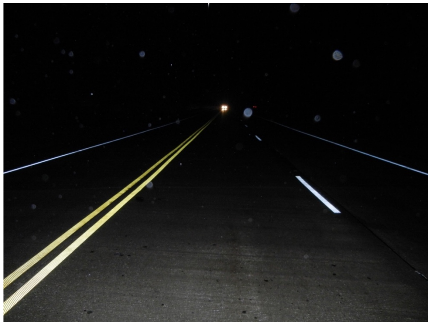
Franklin County; US 127; Recessed Wet-Reflective Tape (Wet Conditions)
