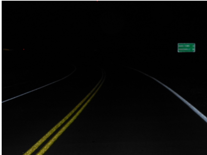
Nelson County; US 31E; Wet-reflective Paint; Surface Applied
