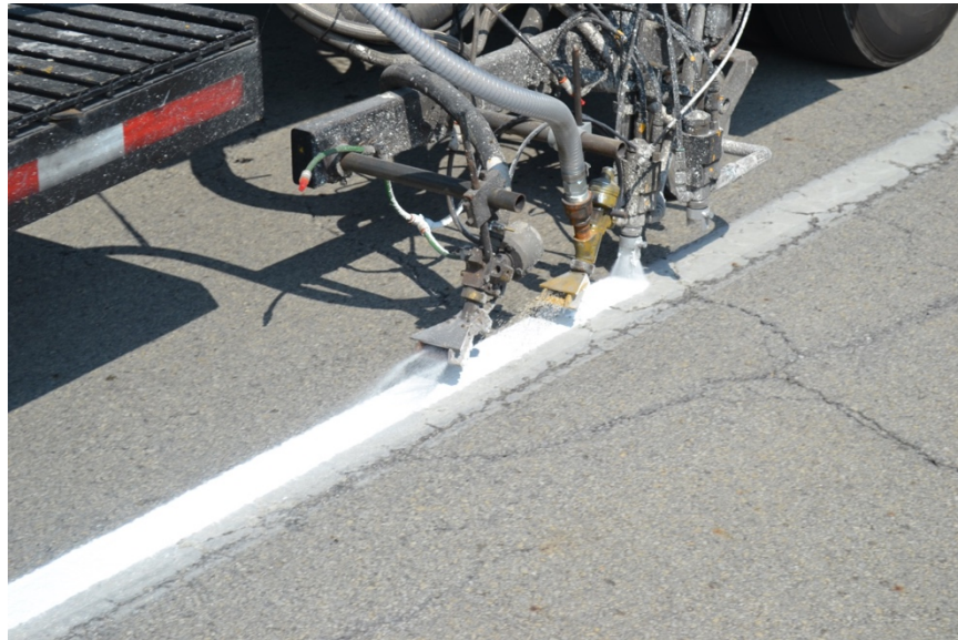
Nelson County; US 31E; Surface Installation of Wet-Reflective Paint
