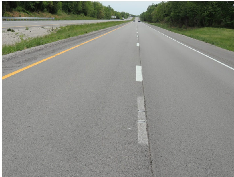
Barren County; Cumberland Parkway; Recessed Markers and Spray Thermoplastic
