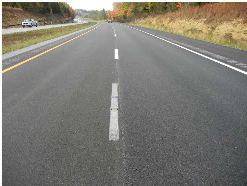
Recessed Marker Installation
