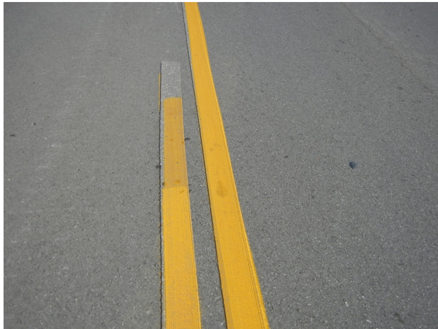
Kenton County; KY 1501; Recessed Wet-Reflective Paint
