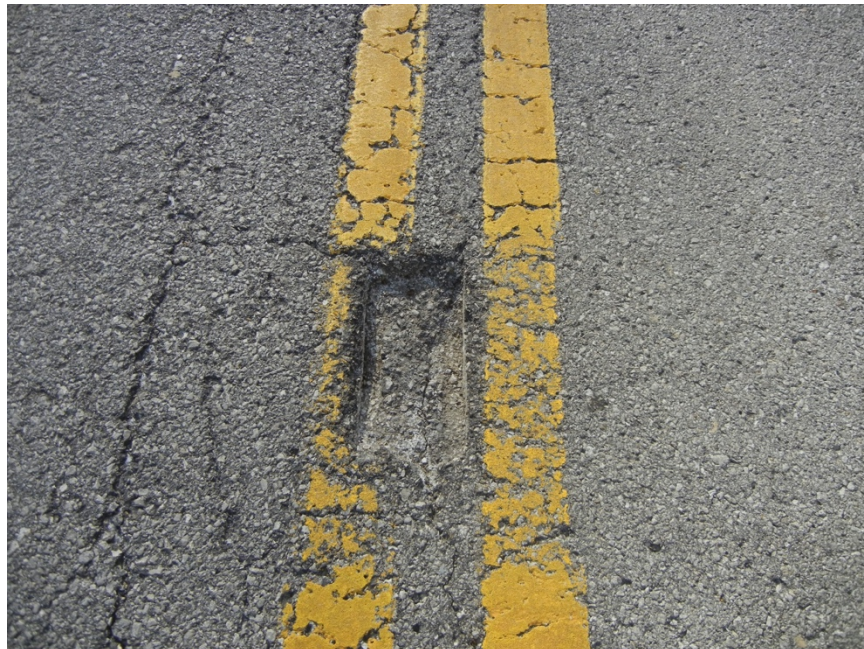
Type V Snowplowable Marker (Durability Issue with Poor Pavement)
