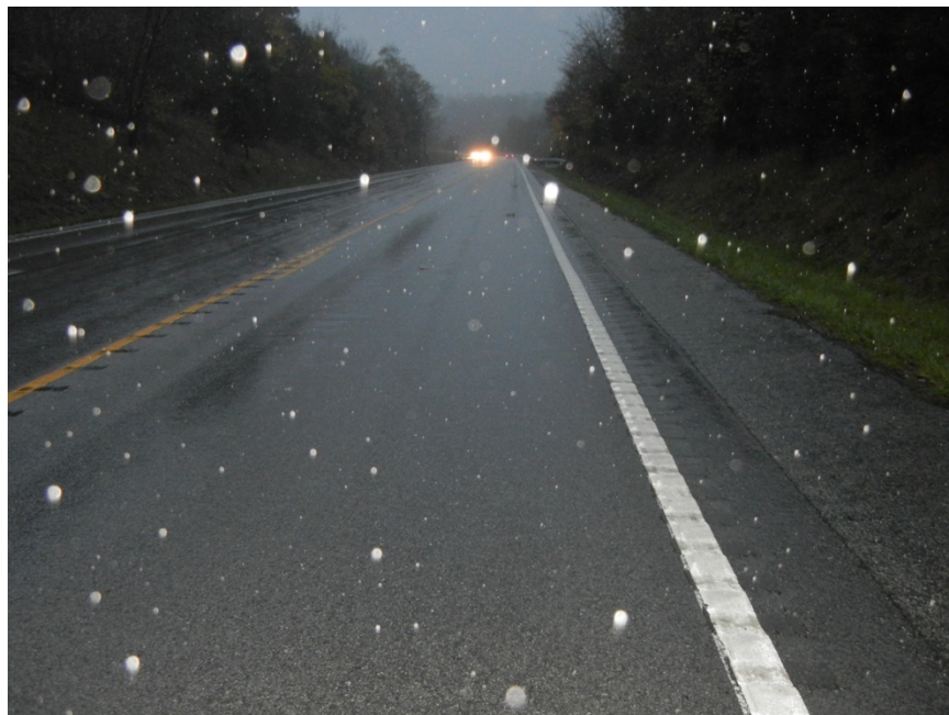
Washington County; KY 555; Ribbon Thermoplastic (Wet Pavement)
