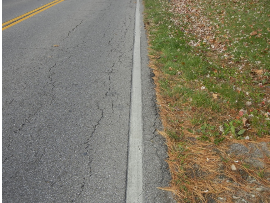
Kenton County; KY 1501; Recessed Wet-Reflective Paint
