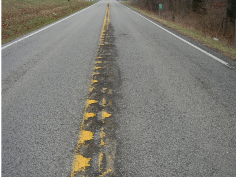
Retrofit Centerline Rumble Strip; Old Pavement
