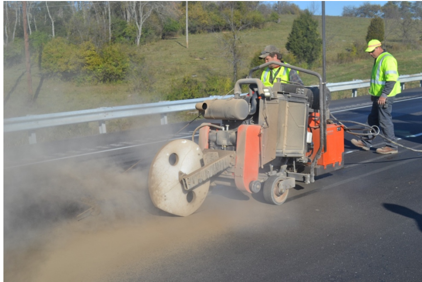
Initial Installation Procedure for Groove for Recessed Markers
