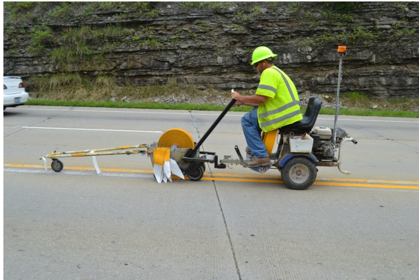
Installation of Wet-reflective Tape in Groove
