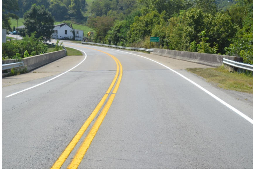
Nelson County; US 31E; Wet-Reflective Paint (Surface Applied)
