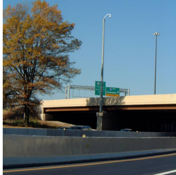
CCTV pole – structure mounted
