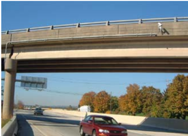
VID Camera mounted on bridge parapet
