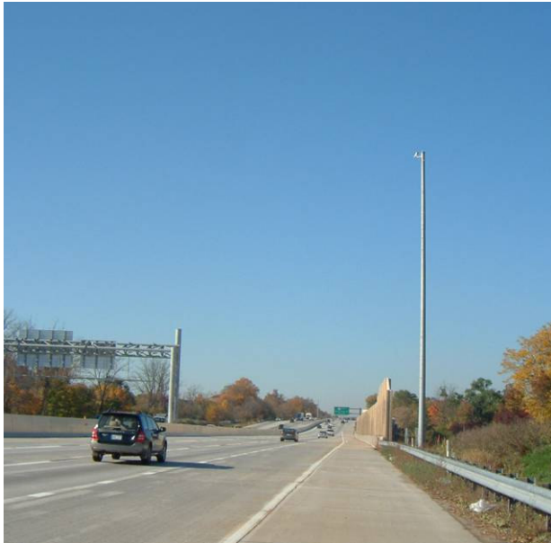
VID Camera mounted on 65-foot pole
