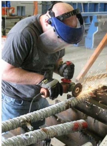
Figure 5.3: Removing Ducts Using Electric Grinder
