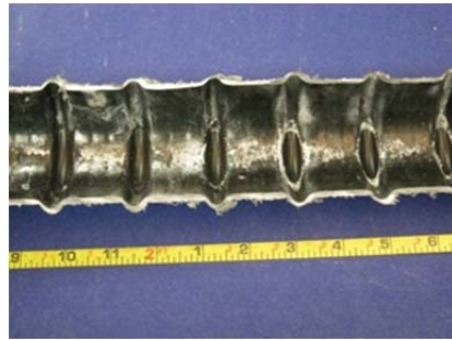
Top of South Duct
