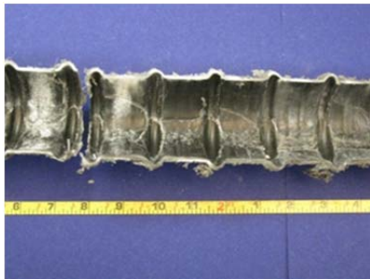
Top of North Duct
