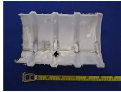
Top of South Duct
