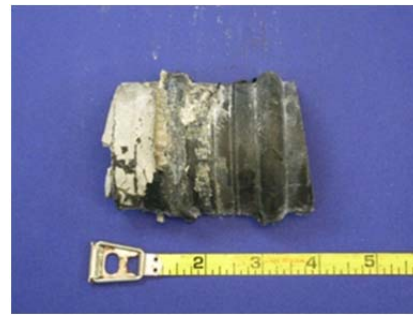
Top of South Duct
