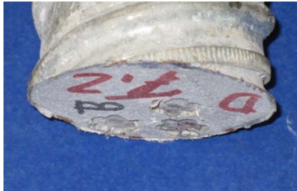
Figure 5.20: Specimen T.2, Debonded Strands in South Anchorage
