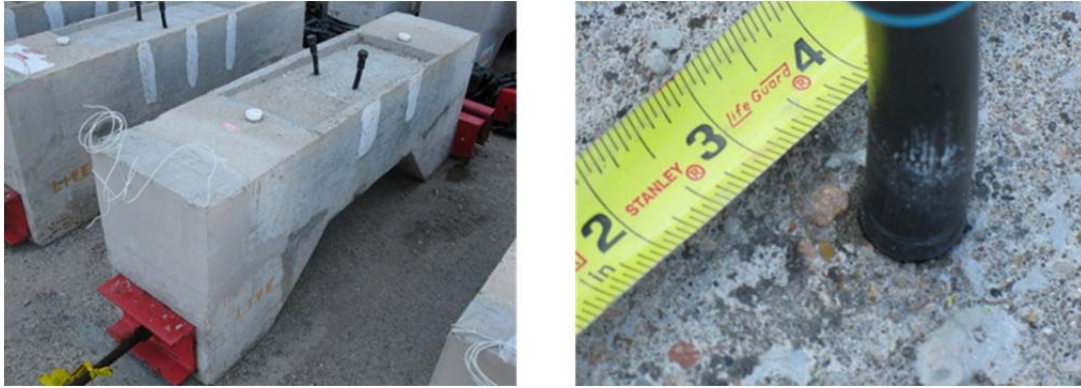
Figure 5.65: Specimen 4.2 Overall (Left) and Discoloration around North Grout Vent (Right)
