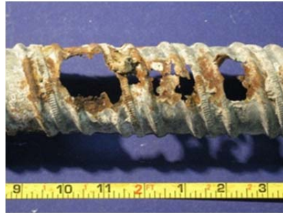
Top of South Duct
