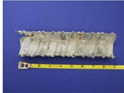
Top of South Duct
