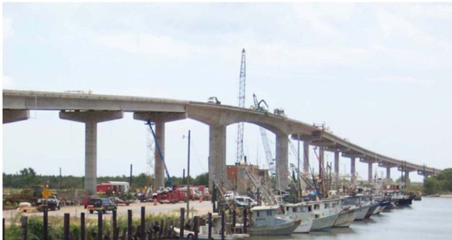
Figure 7.1: FM 2031 Bridge over Gulf Intracoastal Waterway in Matagorda, Texas 25
