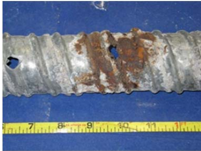
Top of North Duct
