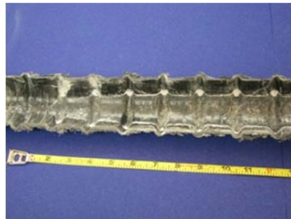
Top of South Duct
