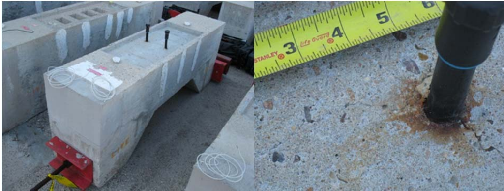
Figure 5.29: Specimen 2.2 Overall (Left) and Corrosion Stains Near Grout Vent (Right)
