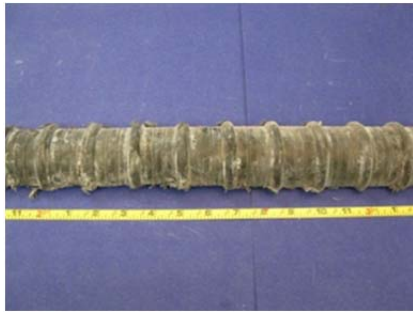
Top of North Duct
