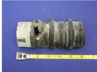
Top of South Duct
