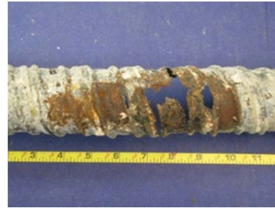
Top of South Duct
