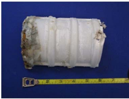
Top of North Duct
