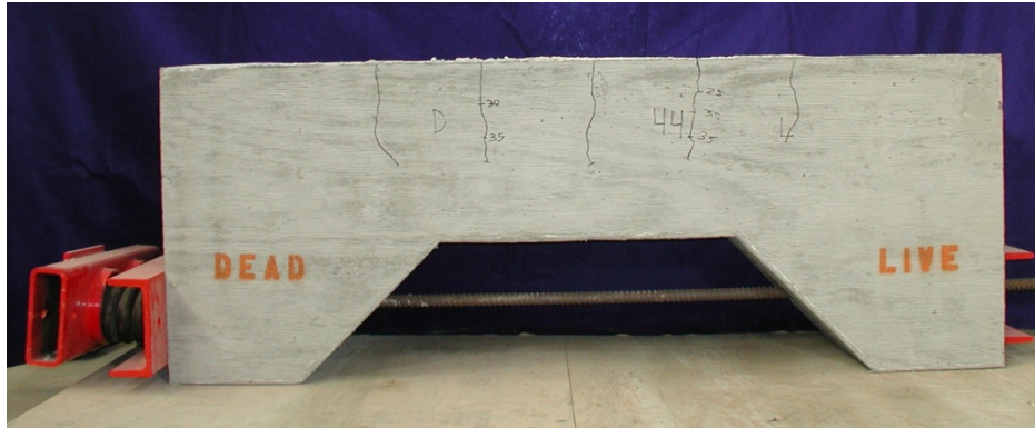
Figure 2.2: Flexural Cracks Occurring in the Reduced Midspan Region 7
