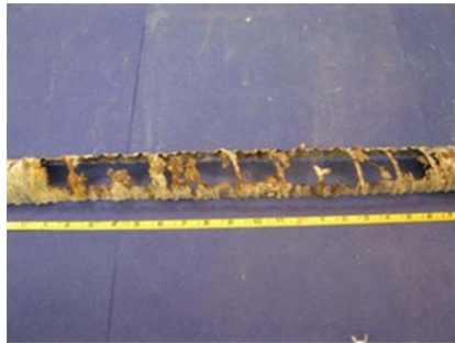
Top of North Duct
