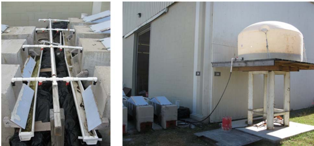
Figure 3.1: Repaired Drippers in Operation (Left) and New Tank System (Right)
