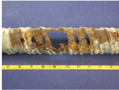
Top of North Duct
