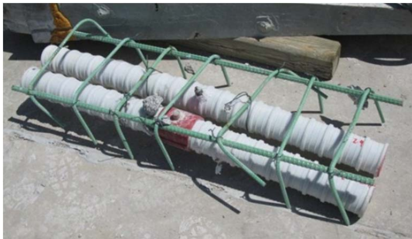
Figure 5.2: Reinforcement Cage and Post-Tensioning Tendons from Specimen 2.4
