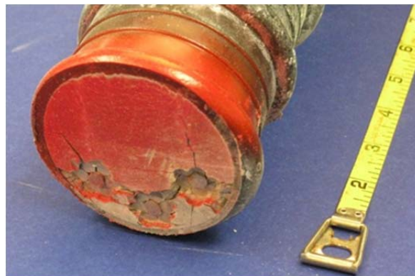
Figure 5.67: Specimen 4.2, Debonded Strands at Live End of South Duct
