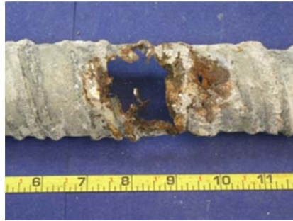
Top of South Duct
