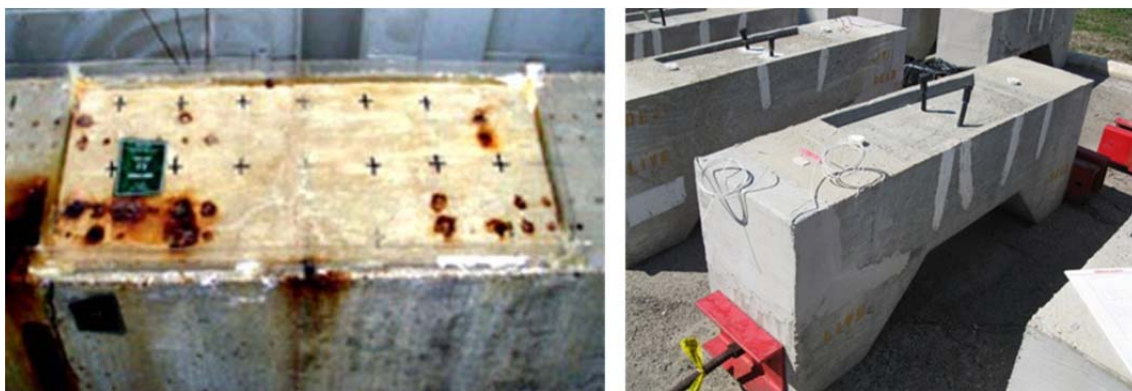
Figure 6.18: Typical Specimen from Project 0-14058 (Left) and Project 0-4562 (Right)
