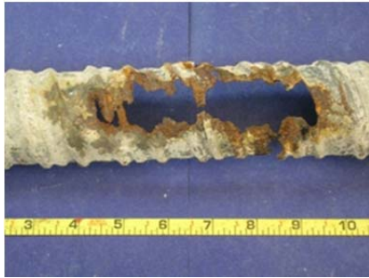
Top of North Duct
