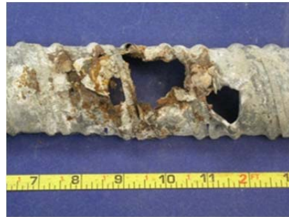
Top of South Duct
