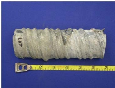
Top of North Duct
