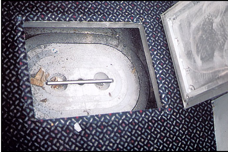
Figure 3-7 Access to “Main Deck” Manhole, Lightning
